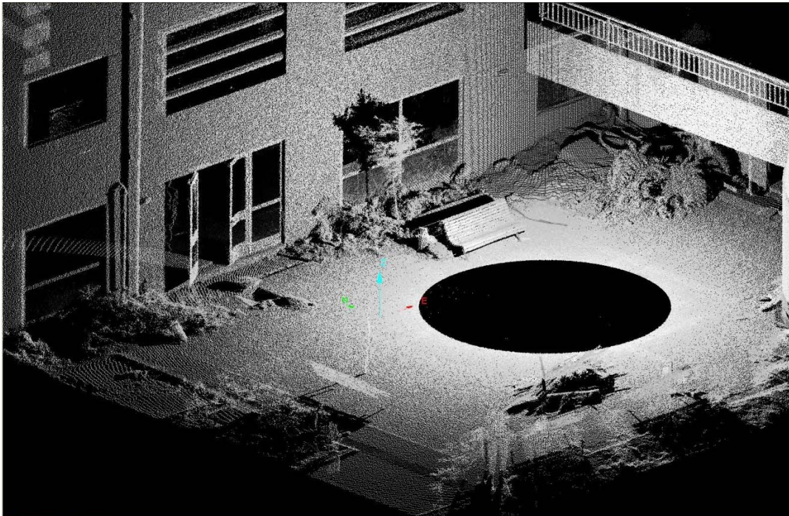
Figure 15.45. Oblique view of the east courtyard of the Provincial Hospital of Curanilahue, 37.47352^{\circ}\text{S} , 73.34824^{\circ}\text{W} . Liquefaction induced structural settlement is clearly evident along the courtyard perimeter.
