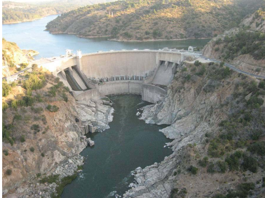
Figure 11.6. March 10, 2010. Rapel Concrete Dam Downstream Face (S34.038754°, W71.590223°)
