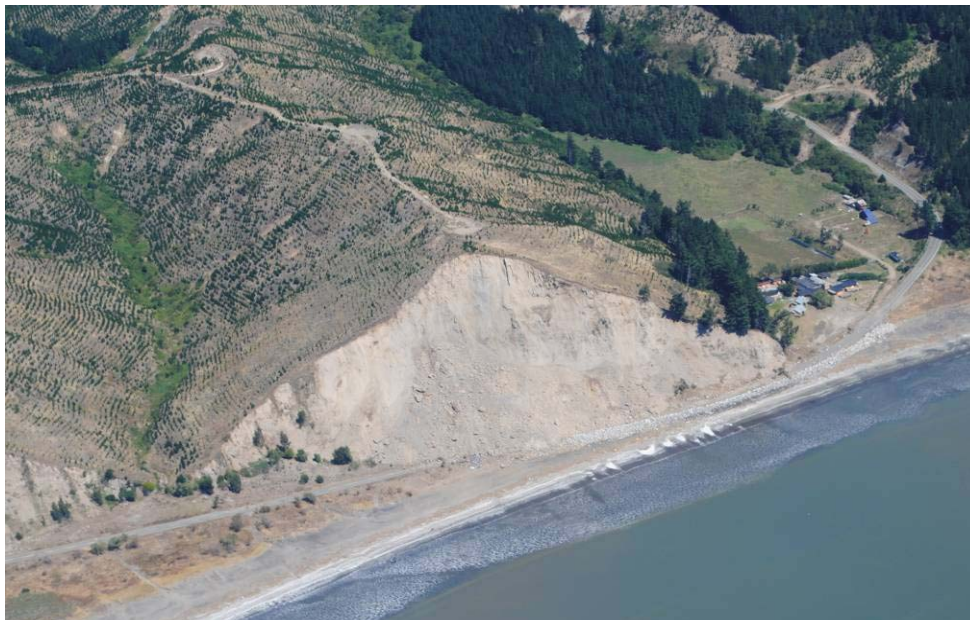
Figure 10.11. Shallow failure along a truncated ridge forcing road closure West of Arauco (37.2437°S, 73.413°W) .
