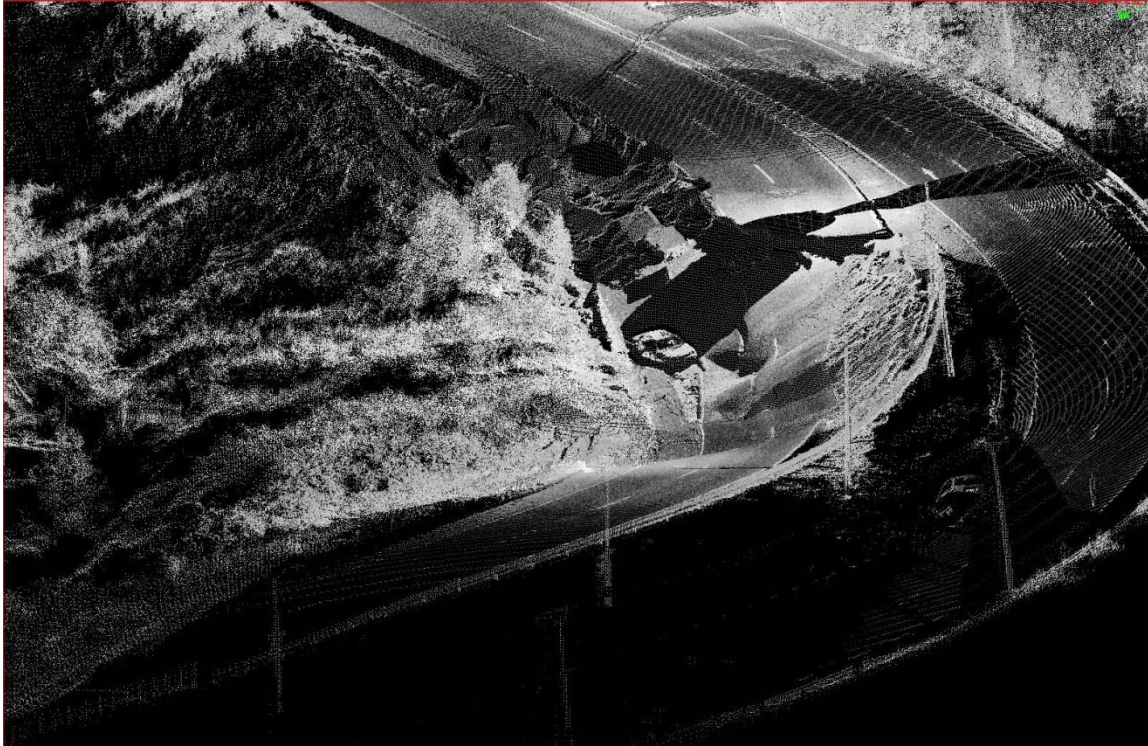
Figure 15.39. Oblique view of route 160 east side embankment failure at the fork in the highway (note vehicle in slide for scale).
