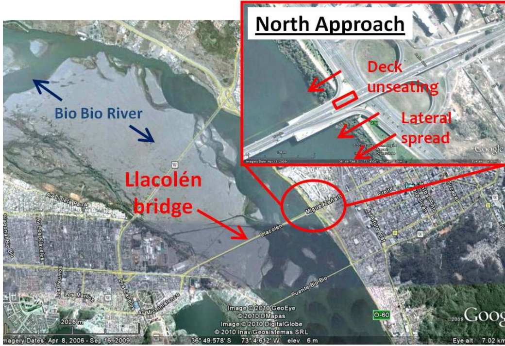
Figure 9.2. Plan view of the Bio Bio river region locating the damaged region of the Llacolén bridge in Concepción (S36.830108°, W73.067991°)
