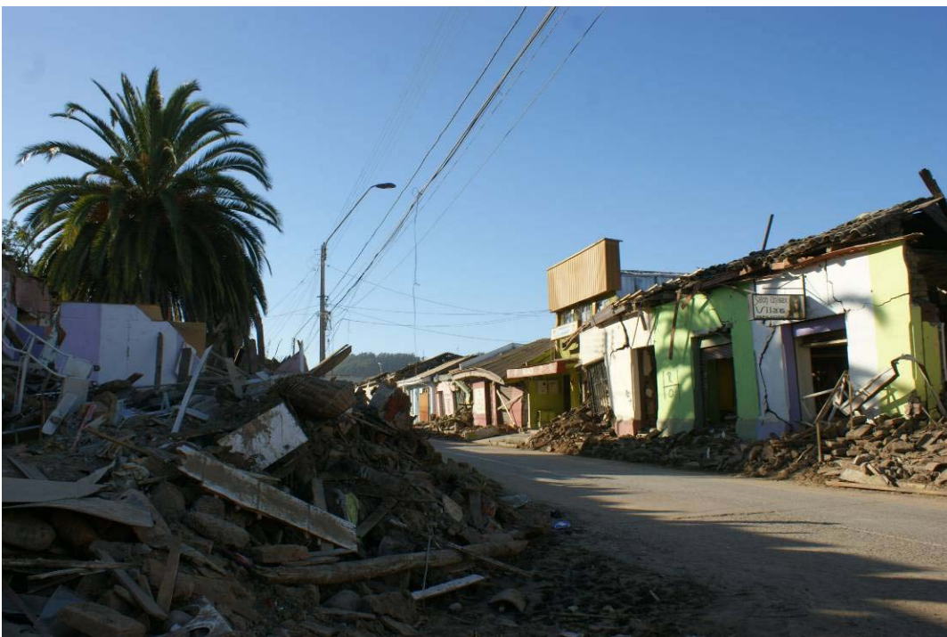
Figure 14.3. Constitucion. Tsunami damage merges with shaking related damage in the older section of the city center with its many adobe and unreinforced masonry buildings. (S35.335383°, W72.410055°; 17:25 hours on 3/15/2010).
