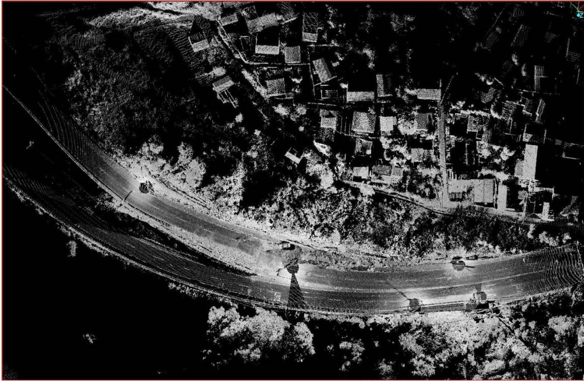
Figure 15.38. Plan view of route 160 embankment failures and neighboring community. One embankment failure is above the fork in the highway, and the second failure is on the lower right side of the merged highways.
