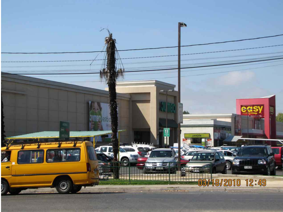
Figure 5.29. Modern (engineered) structures adjacent to the river that showed no or minor damage (S 35.437897° W 71.660151°, 1249 hrs on 03/18/2010).
