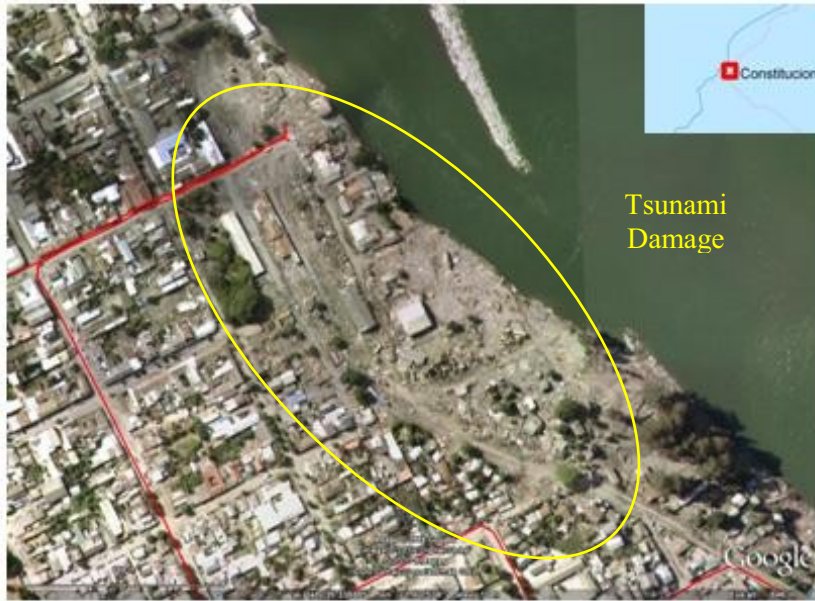
Figure 3.29. Pre/Post Imagery of Constitución (35.337° S, 72.403° W)
