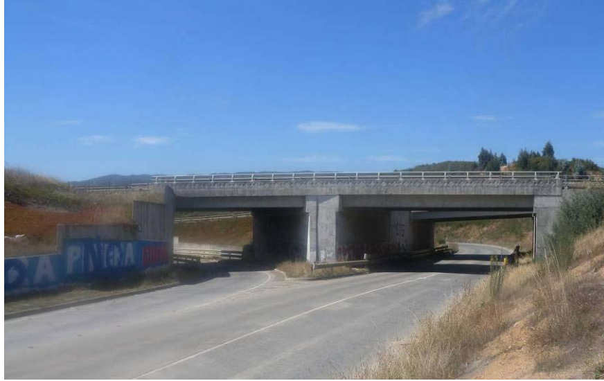
Figure 12.5. Multiple retaining structures for highway overpass structures south end of Coronel (37.0455°S, 73.1421°W)
