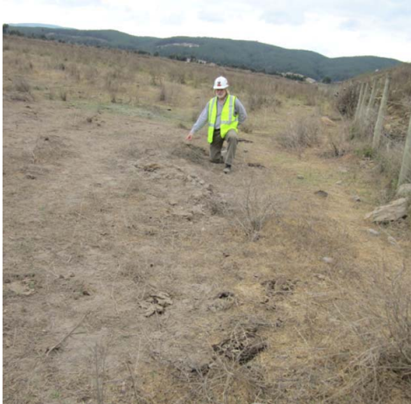
Figure 15.68 Compression ridges at toe of embankment, due to liquefaction of underlying soil and settlement of embankment, north abutment of the bridge, Puente Mataquito, 35.050712°S, 72.162258°W, April 16, 2010.
