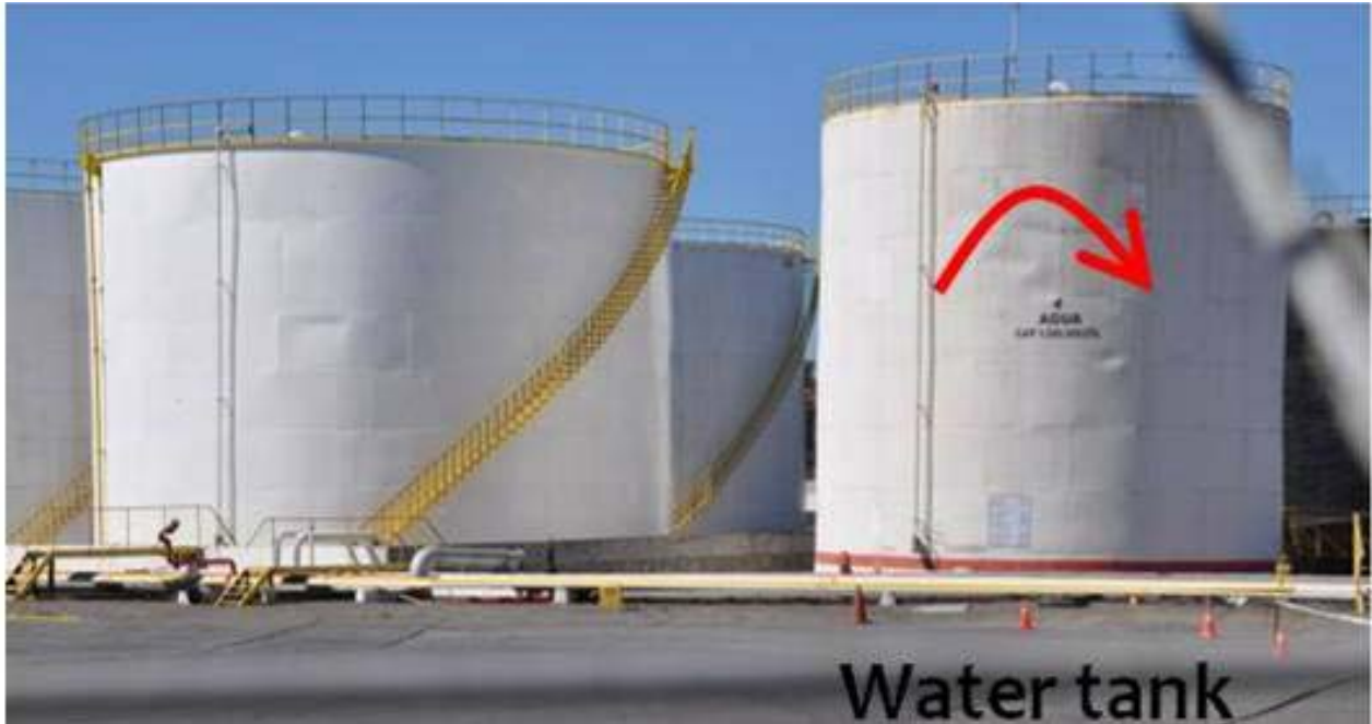
Figure 8.30. Tilted water tank at Petrobras gas facility (S36.7270°, W73.1272°; 1250 hrs, 03/15/2010).
