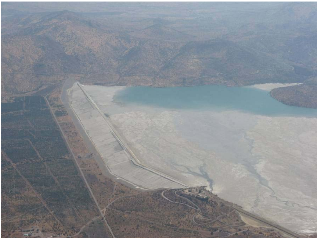
Figure 11.8. March 10, 2010 View of Ovejeria Tailings Dam from Helicopter (S33.054182°, W70.768953°)
