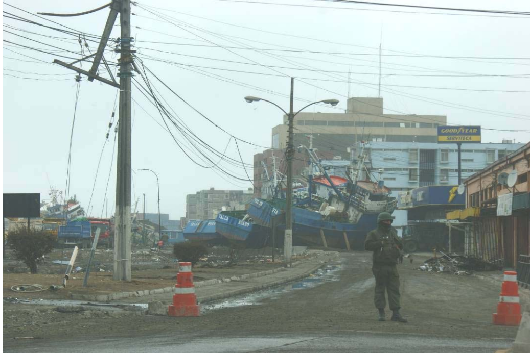
Figure 14.6. Tsunami damage near Navy facilities and bayside port of Talcahuano. (S36.711305°, W73.114808°; 12:39 hours on 3/16/2010)
