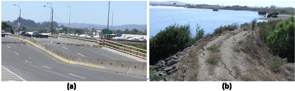
Figure 9.10. Juan Pablo II northeast approach: (a) Settlement of bridge deck near bridge approach (S36.815900° W73.084064°; 1455 hrs on 3/15/2010), (b) Lateral spreading on northeast bridge abutment.
