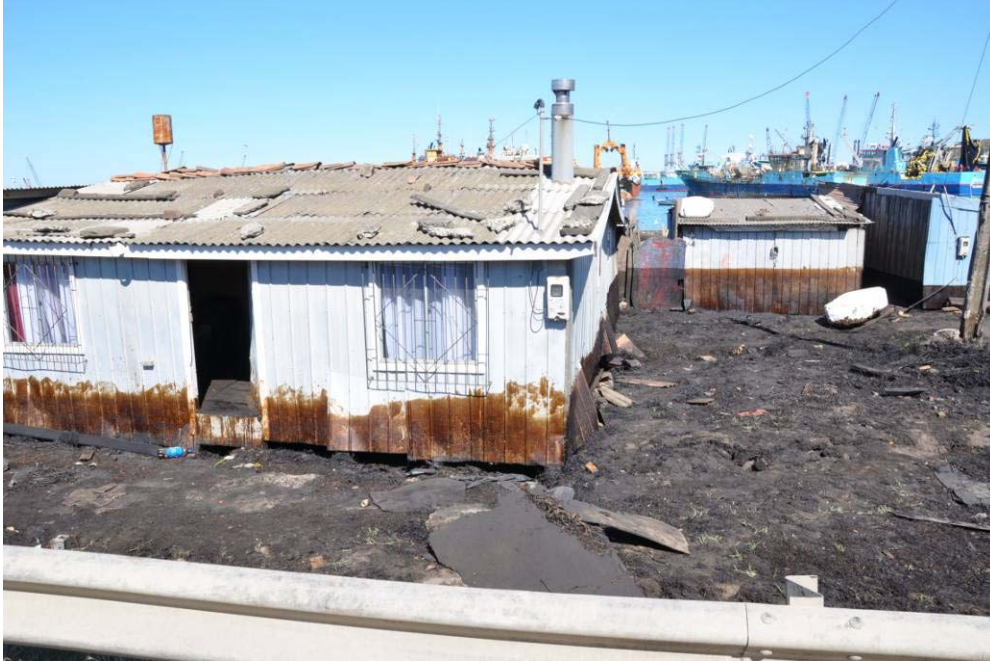
Figure 8.28. Evidence of water level rise at port area – neighboring fish packaging facility (S36.7267°, W73.1282°; 1200 hrs, 03/15/2010).
