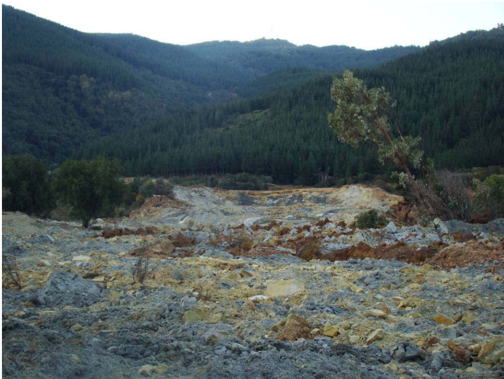
Figure 11.26. March 11, 2010. View Along Flowpath of Tailings (35.18468° S, 71.759410° W)
