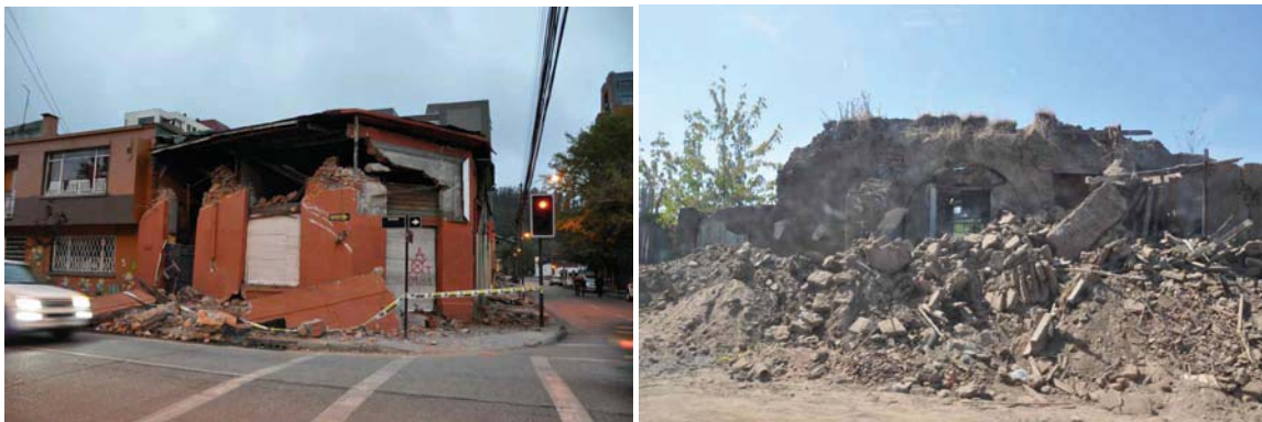
Figure 5.28. Adobe and unreinforced concrete damage concentrated adjacent to the Maule river across Talca (pictures shot from passenger seat while driving).
