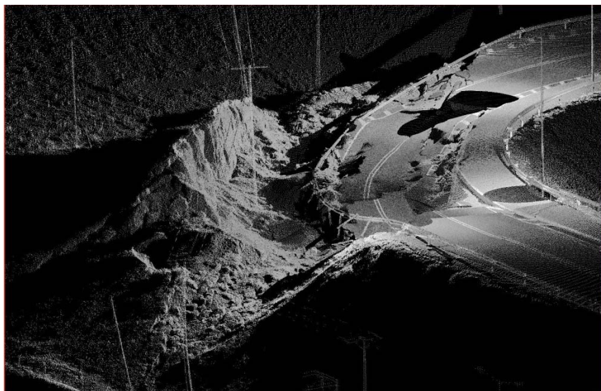
Figure 15.48. Closeup of the Route 5 overpass embankment failure from the southeast side. The embankment along the outside curve can be seen to have slid out laterally 16m into the field.
