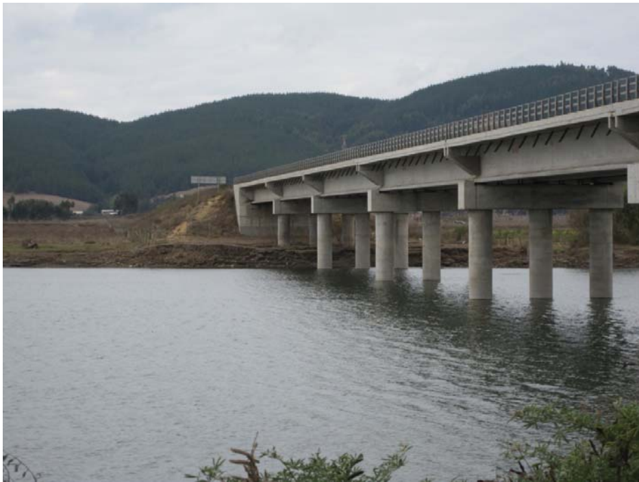
Figure 15.65 Lateral spreading on the north end of the bridge, Puente Mataquito, 35.050712°S,72.162258°W April 16, 2010.
