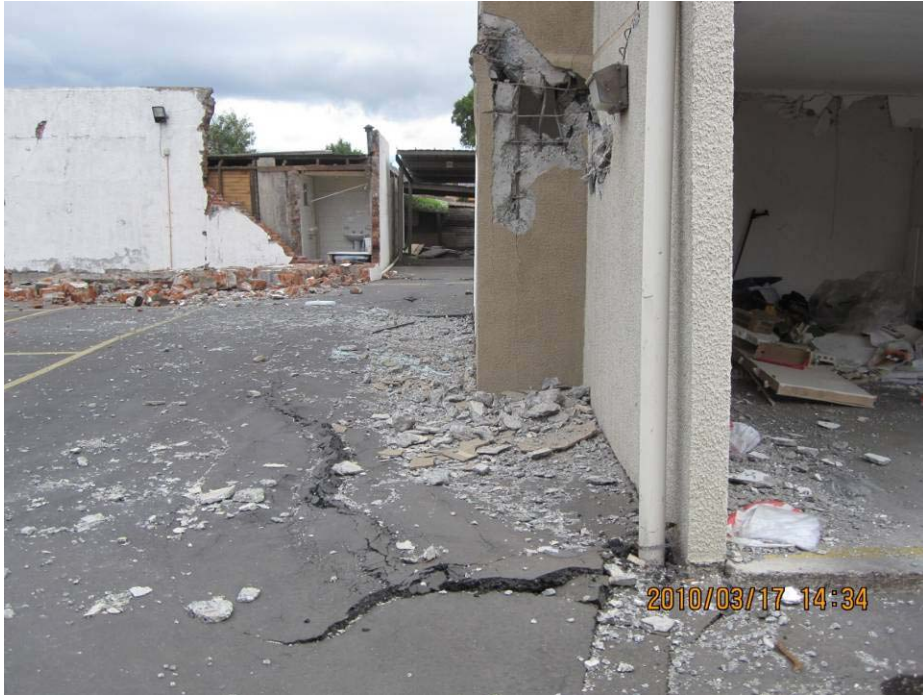
Figure 7.38. Pavement buckling on south side of south wing, view looking west (S36.8205°, W73.0619°; 03/17/10).
