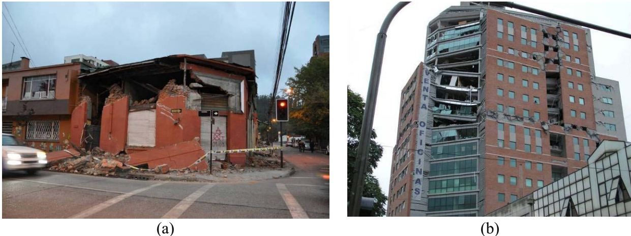
Figure 7.1. (a) Typical construction type and observed damage within the city of Talca ( S36.8323^\circ, W73.0554^\circ ; 1230 hrs on 3/18/2010) and (b) Significant structural damage, including partial collapse of a floor, of a modern high-rise building in downtown Concepción ( S36.8296^\circ W73.0550^\circ ; 2000 hrs on 03/17/2010).
