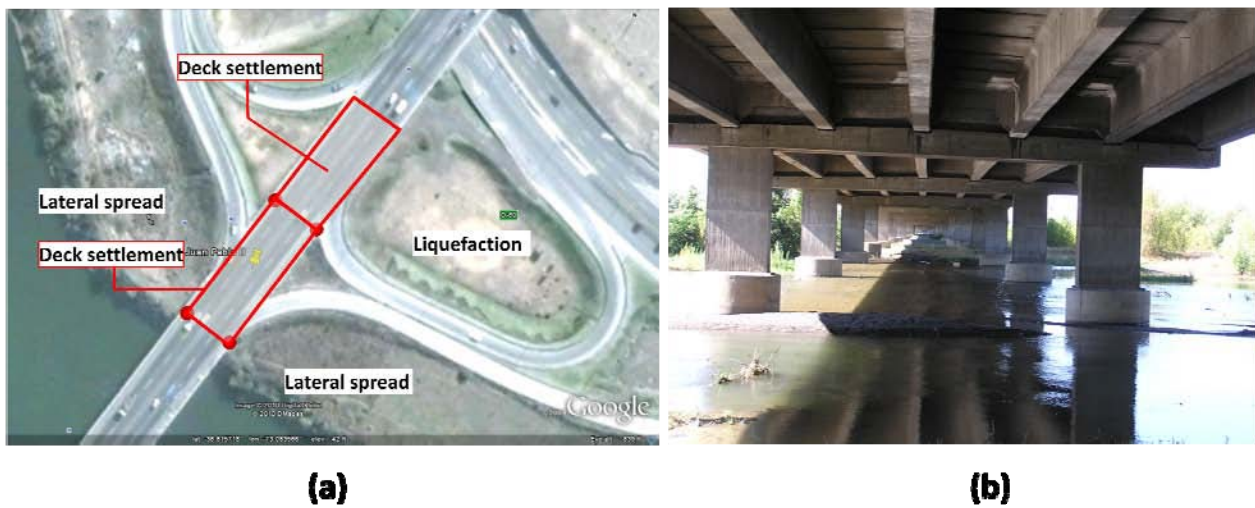
Figure 9.9. Juan Pablo II Bridge (a) Google Earth view of northeast Approach with schematics of observed damage (S36.815864° W73.083674°) (b) Typical bridge bent configuration (S36.828181° W73.095850°; 1636 hrs on 3/15/2010).
