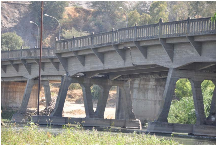
Figure 9.34. Deck unseating and shear failure of longitudinal spanning girders of the Talca pedestrian bridge at the vista area (S35.421044, W71.683197; 1354 hrs on 3/18/2010)
