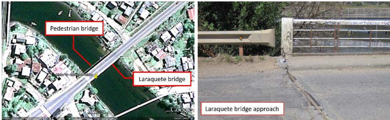
Figure 9.46. Laraquete bridge (a) Aerial view (S37.166788° W73.184486°), (b) Bridge approach (S37.166804° W73.184760°; 1430 hrs on 3/10/2010)
