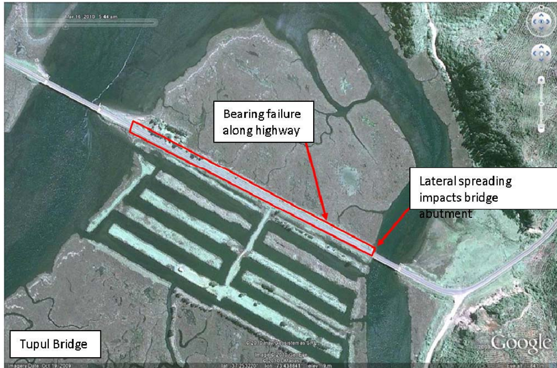
Figure 9.50. Damage to roadway and bridge due to ground failure near town of Tubul, Chile (S37.254345°, W73.437021°).
