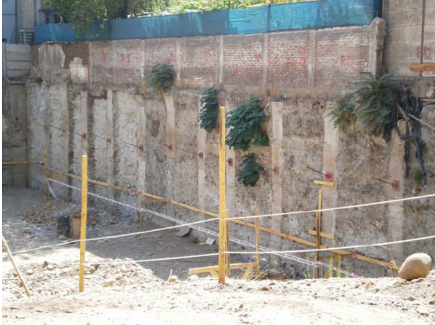
Figure 12.11. Undamaged temporary retaining structure in Santiago.
