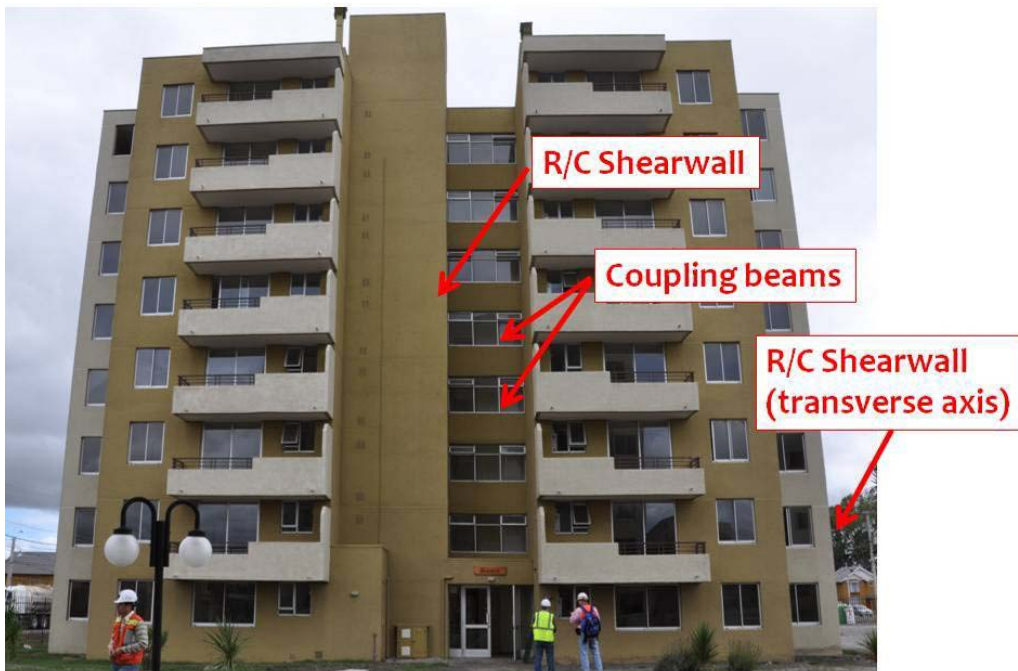
Figure 7.18. Elevation of the Riesco building depicting the general components of the structural system of the building (image taken at S36.790929°, W73.081296°; 1400 hrs on 3/17/2010).
