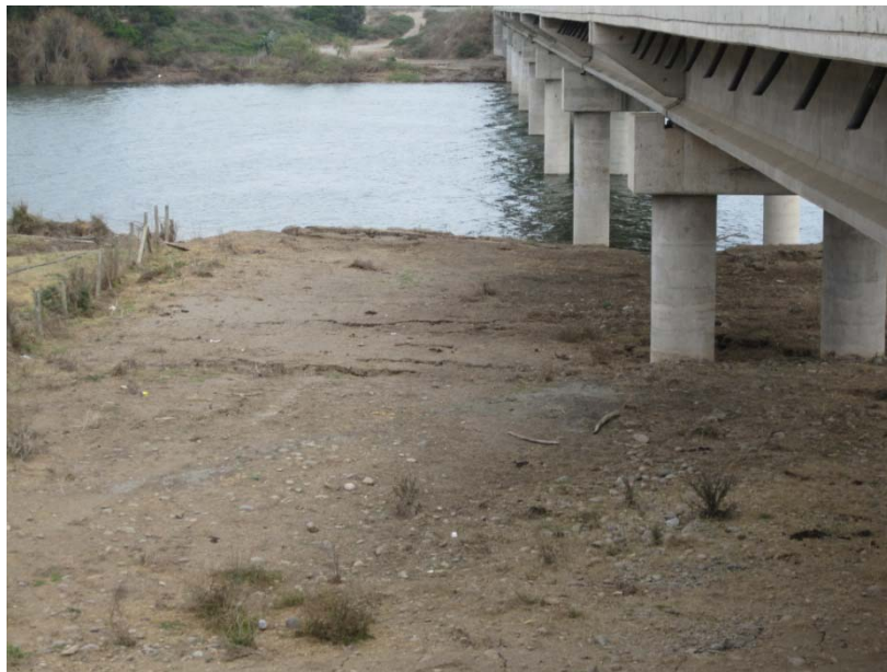
Figure 15.69 Lateral Spreading towards the river, north abutment of the bridge, Puente Mataquito, 35.050712°S, 72.162258°W, April 16, 2010.
