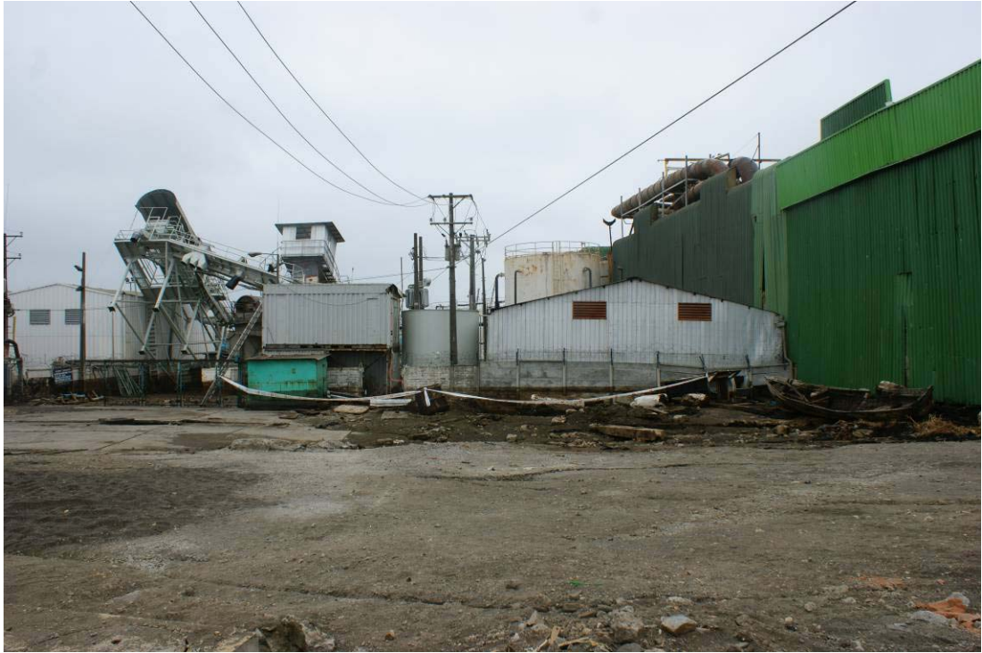
Figure 14.16. Port San Vicente, Talcahuano. The damaged Concesion Maritima fish processing plant. (S36.725892°, W73.128678°; 11:50 hours on 3/16/2010)
