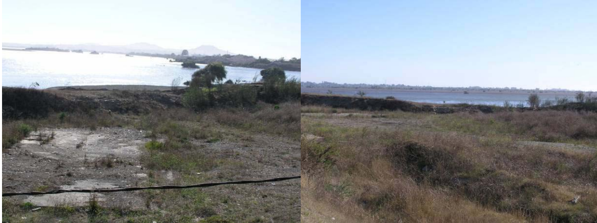
Figure 11.37. View obliquely down on the slumped levee from the NE approach of the Juan Pablo II bridge with evidence of sand ejecta in the foreground, and ground level view looking back at slumped level crest (S36.814555°, W73.084624°); 1700 hrs on 3/15/10).
