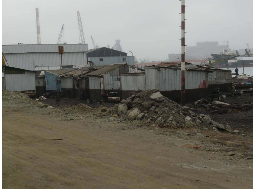
Figure 13.6. One-meter high dark stains on buildings at Talcahuano port facilities along Bahia San Vicente mark the elevation of the tsunami. Major damage of port facilities, including a fish processing plant were caused by a combination of factors, including modest tsunami inundation in areas that dropped vertically due to liquefaction-induced lateral spreading (S36.727076° W73.128058°, 1258 hrs on 03/16/2010).
