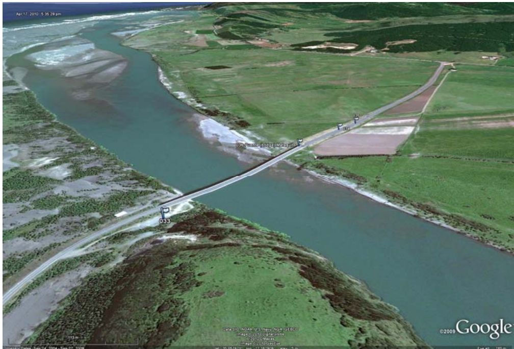
Figure 15.63 Puente Mataquito, looking north, 35.050712°S,72.162258°W, April 16, 2010.
