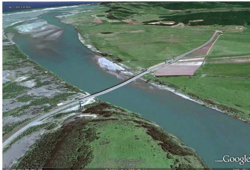
Figure 9.38 Puente Mataquito, looking north, S35.050712°,W72.162258°, April 16, 2010
