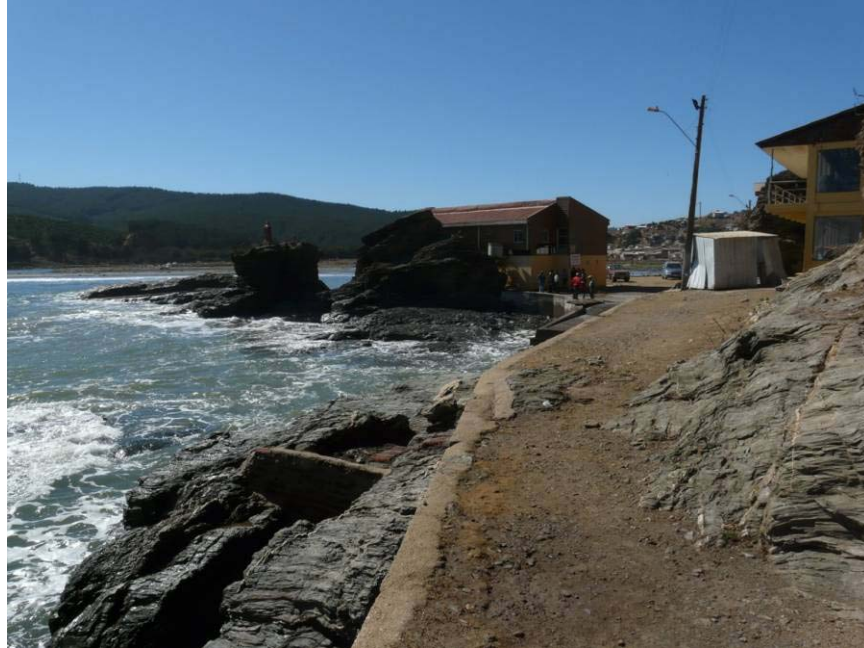
Figure 4.25. The shoreline at Bucalemu has shifted over 25 m east as a result of tsunami erosion and, possibly, coseismic subsidence. Pre-earthquake imagery shows a 25-m-wide sandy beach west of the boat ramp and sea wall that is now under attack by ocean waves. Where waves now crash on rocks in this photo taken two weeks after the earthquake, once was a wide sandy beach before tsunami flooding. (S34.639916° W72.044664°, 1142 hrs on 03/15/2010).
