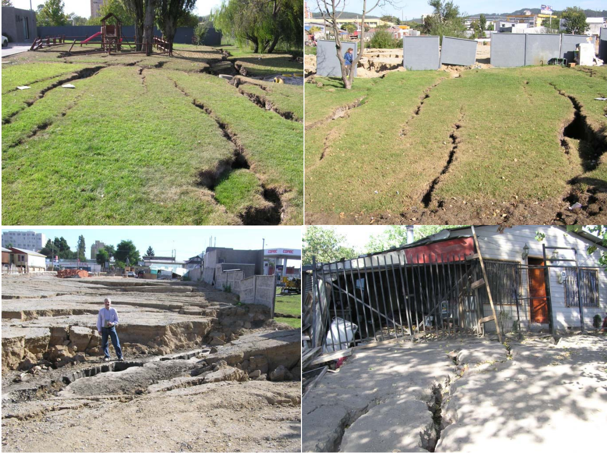
Figure 6.8. Effects of the lateral spread in Concepcion at the southwest edge of Laguna Las Tres Pascualas (S36.8153°, W73.0458°; 1700 hrs on 3/14/2010).
