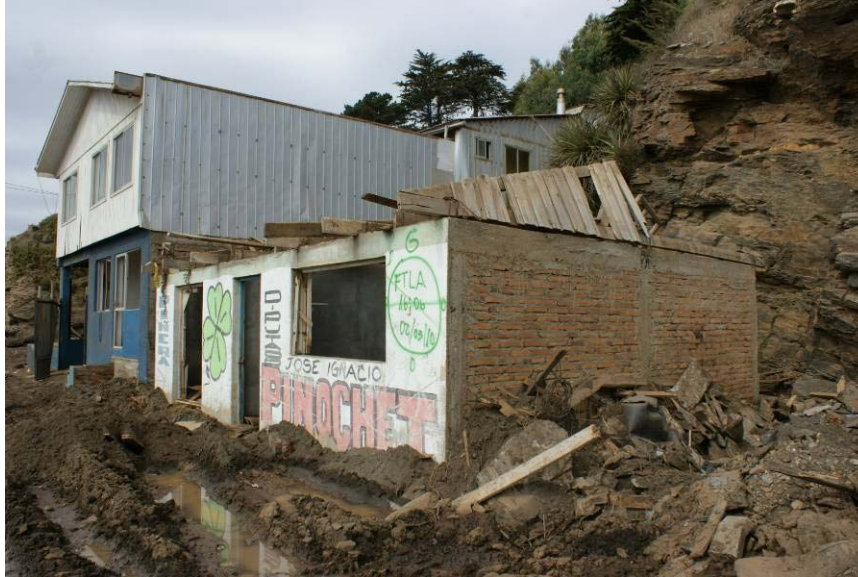
Figure 13.22. The blue and white two-story house in the beach community of El Torreon was heavily damaged by the tsunami and all but the walls of the adjacent vacation house was destroyed. The tsunami arrived at 4:05 am, about 30 minutes after the earthquake, and the water remained high for four hours when it started to retreat around 8 am (S35.8215°, W72.5990°, 03/17/2010).
