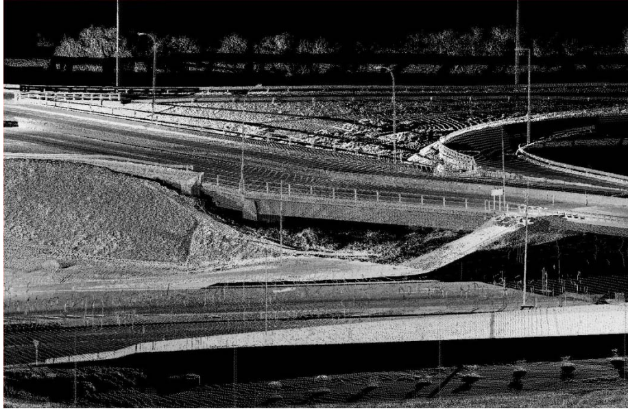
Figure 15.23. Settled bridge pier at the approach embankment of the Juan Pablo II Bridge (S36.815864°; W73.083674°).
