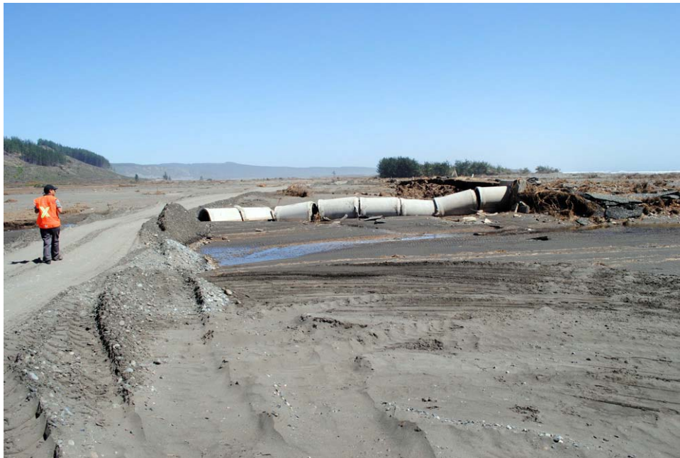
Figure 4.21. Ground photograph of area inundated and scoured by tsunami between Rio Mataquito and the town of Putú. Sections of concrete pipe were exposed and highway asphalt was eroded by tsunami flow, suggesting very high velocities; the extensive inundation in this area suggests possible land subsidence. (S35.115414° W72.203106°; 1500 hrs on 03/08/2010)
