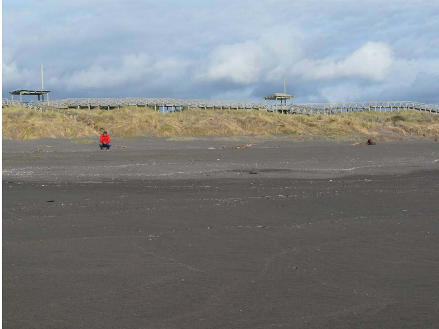
Figure 13.24. The tsunami carried wood and debris about halfway up these dunes near Chanco but left the walkway along the dune crest undamaged (S35.739239° W72.571586°, 1829 hrs on 03/17/2010).
