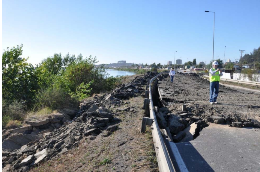
Figure 9.23. Damage to the approach road north of the La Mochita Bridge (S36.846473°, W73.055881° on 3/15/2010). View looking north. The Bio Bio river is shown on the left (west) of the view.
