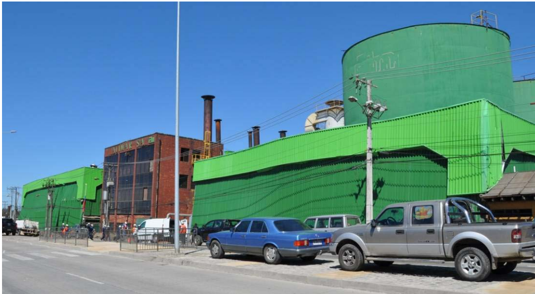
Figure 8.23. Damage to fish packaging facility (S36.7260°, W73.1288°; 1356 hrs, 03/15/2010).
