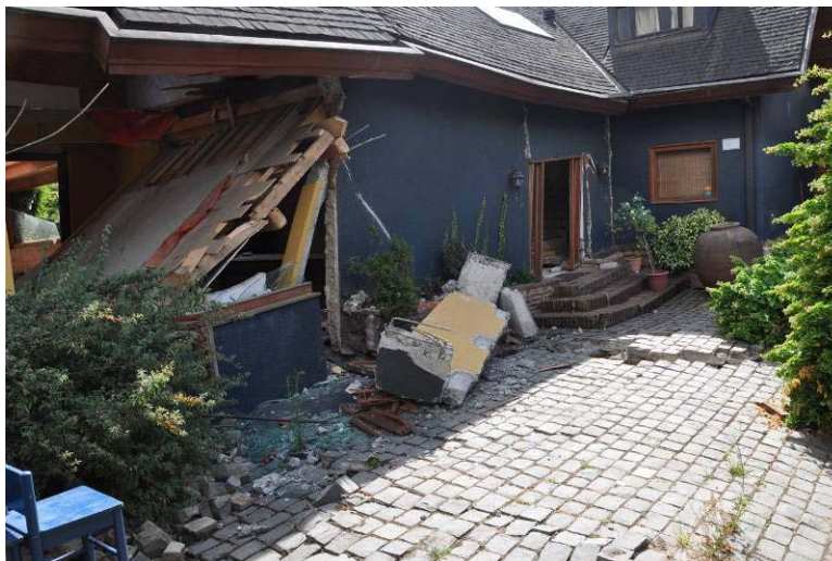
Figure 7.34. Single family residence severely damaged at backside of scarp (S36.79108°, W73.05728°; 1200 hrs on 3/17/2010).
