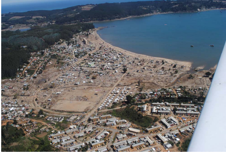
Figure 4.16. Aerial view looking west of town of Dichato, showing tsunami damage focused on north-facing shoreline in Bahia Talcahuano. (S36.548022° W72.922225°; 1301 hrs on 03/09/2010)
