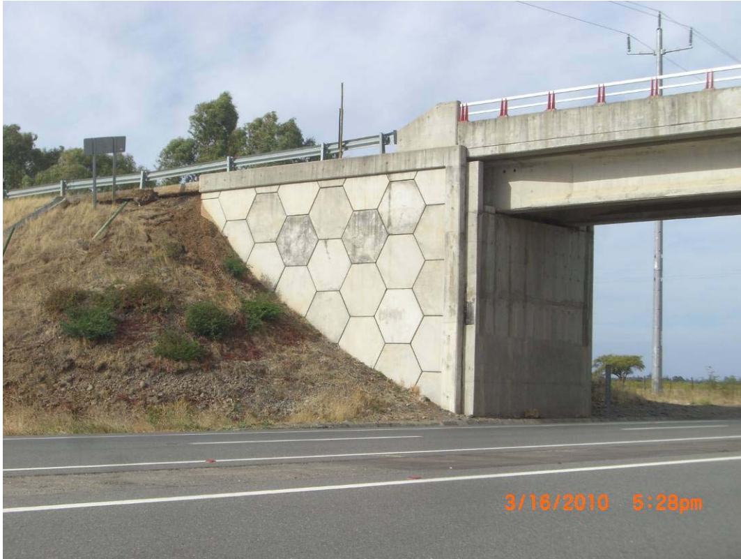
Figure 12.4 Undamaged MSE wingwall on overpass structure over highway 152 west of Chillan despite sliding of adjacent fill slope (S36.6588, W72.2776).
