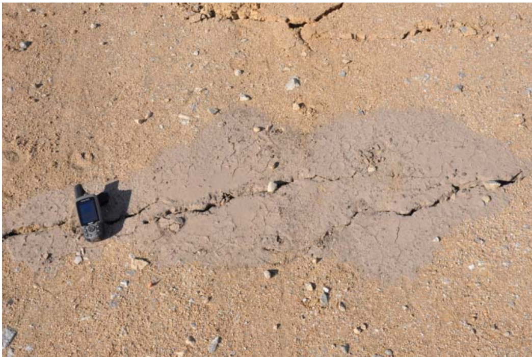
Figure 6.7. Liquefaction boils in undeveloped land area along west shore of Tres Pasuales lagoon in Concepcion (S36.8155°, W73.0460°; 3/14/2010)
