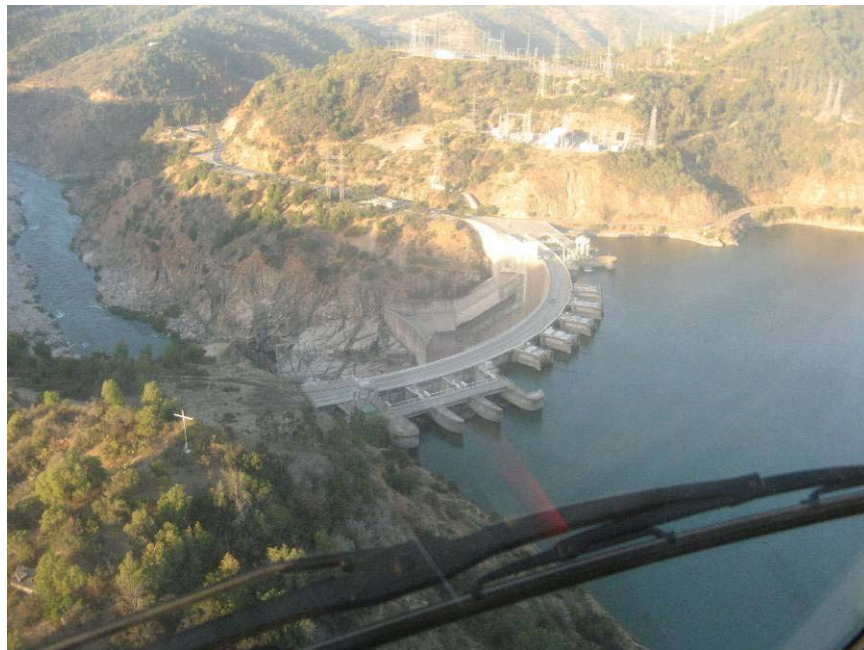
Figure 11.7. March 10, 2010 – View of Upstream of Rapel Concrete Dam (S34.043786°, W71.592053°)
