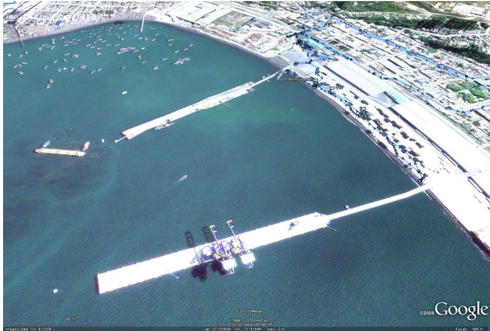
Figure 15.73 Port Coronel, area marked by GPS tracks along the coast experienced lateral spreading ( 37.028874^{\circ}\text{S} , 73.149768^{\circ}\text{W} ).
