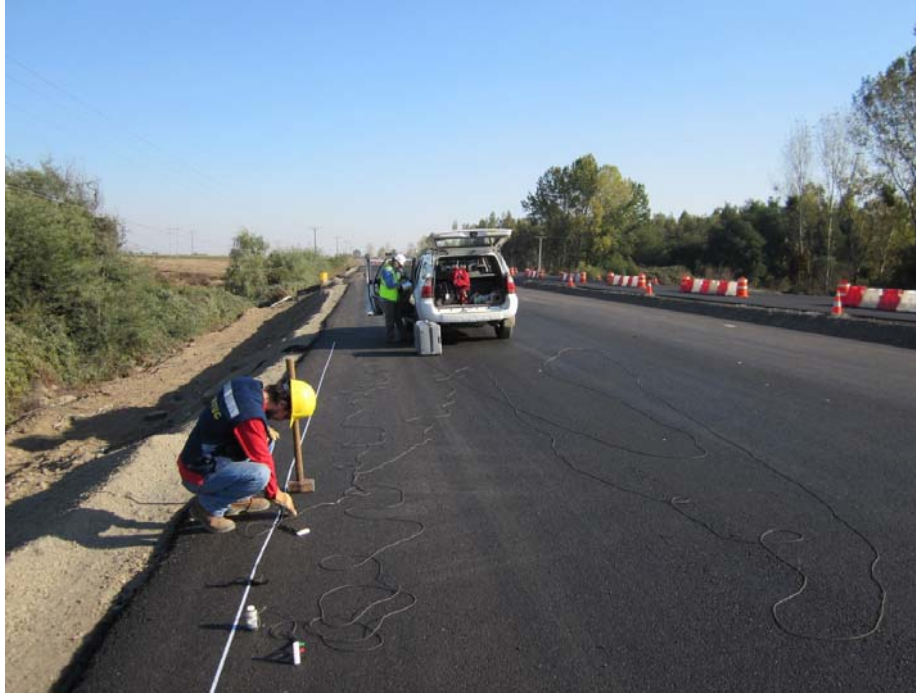
Figure 15.81 SASW line, North bound lane looking south, Roadway Embankment ~5km south of Parral, Ruta 5 Sur, April 15, 2010 (-36.185671°S,-71.825415°W).
