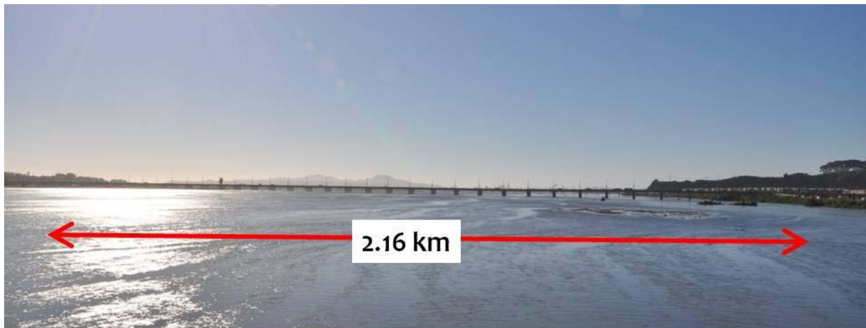
Figure 9.3. Elevation photograph of the Llacolén bridge in Concepción (S36.830108°, W73.067991°).
