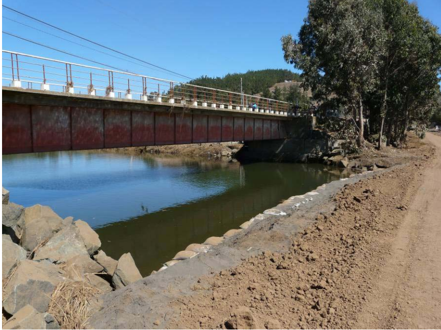
Figure 13.26. Debris clinging to the railing of this damaged bridge in Pichibudi suggests minimum tsunami flow depths reached 5.15 m. Local residents reported flow depths of 6.65 m above the creek. Anecdotal accounts suggest the tsunami moved a bus 80 m up the creek valley. Tsunami damage along coast becomes heavier toward the south of this site in Iloca (S34.880055° W72.155819°, 1515 hrs on 03/15/2010).
