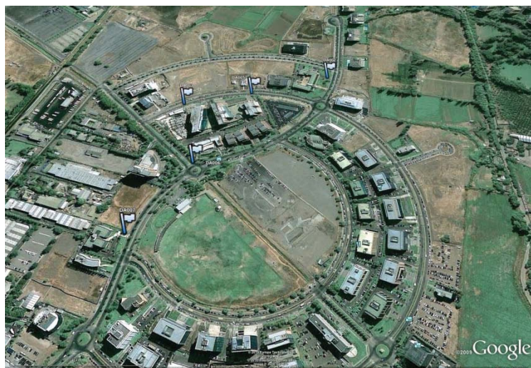
Figure 5.9. Aerial view of Ciudad Empresarial, depicting the structures that were inspected during reconnaissance.
