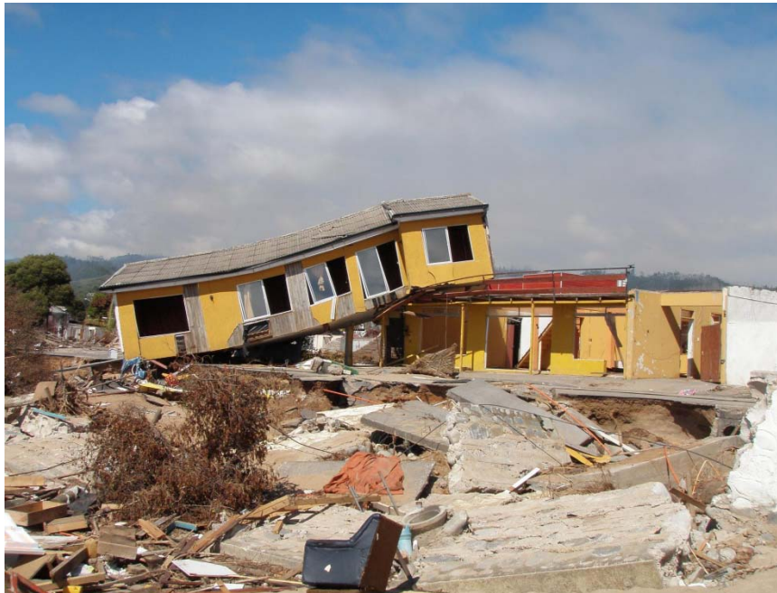
Figure 13.18 The tsunami wave removed the lightweight wooden second story of this house from its more substantial masonry and concrete block first floor (S36.546 , W72.935 , 2010 hrs, 3/13/10).
