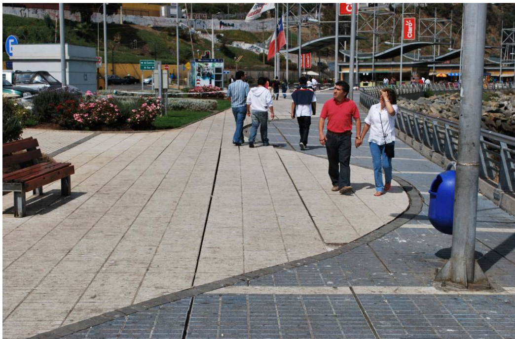
Figure 8.32. Cracks on brick pavement behind quay wall in San Antonio Port (S33.5830°, W71.6138°; 1432 hrs, 03/14/2010).
