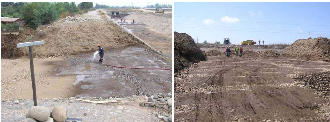
Figure 11.36. Site of earthen levee breach during reconstruction on March 18, 2010 ( S35.698672^\circ , W71.487294^\circ ).
