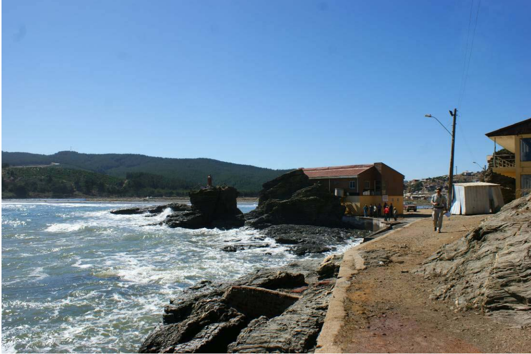
Figure 14.10. Bucalemu. Waves crashing up against the pub building. The cement boat launch ramp and former beach are now submerged after the tsunami. (S34.474325°, W72.023918°; 10:42 hours on 3/15/2010)
