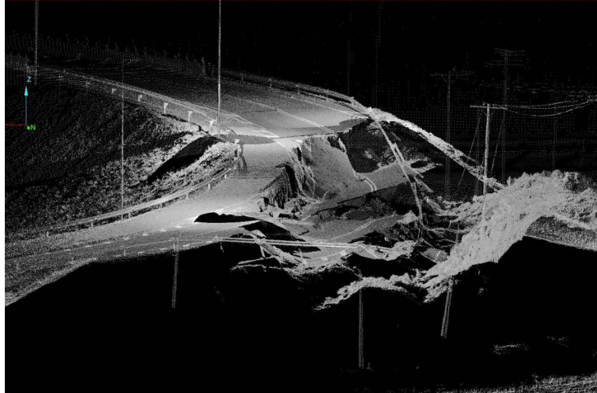
Figure 15.49. Oblique view of the Route 5 overpass embankment failure from the northwest side. Much of the roadbed slumped into the graben left behind as the outside slid out laterally to the southwest.
