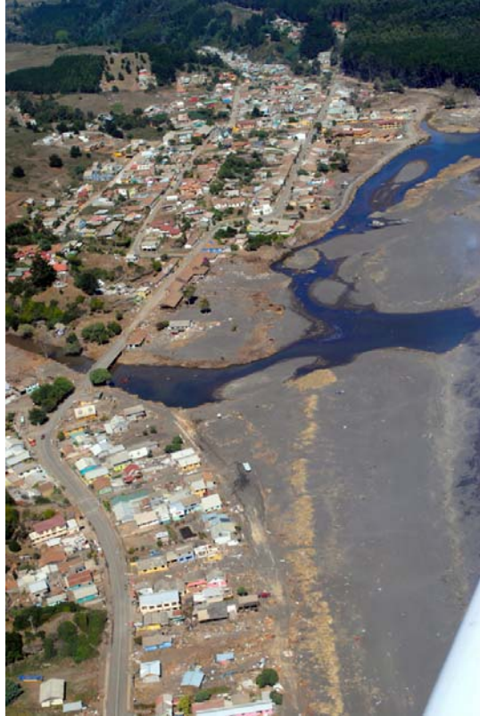
Figure 4.19. Aerial view looking south at village of Curanipe, including evidence of tsunami damage (i.e., red truck beneath bridge). Field observations of wave-cut platforms in this area indicate earthquake-related uplift of approximately 2 m. (S35.843297° W72.631214°; 1225 hrs on 03/09/2010)
