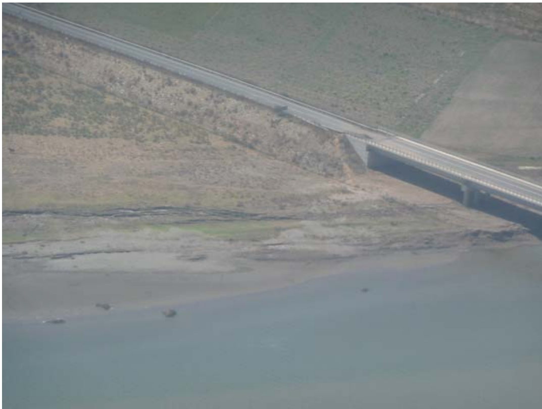
Figure 6.10. Lateral spreading on the north bank of the Mataquito Bridge along the coastal highway (S3505078 °, W72.16240°, 11:00, 3/10/10).
