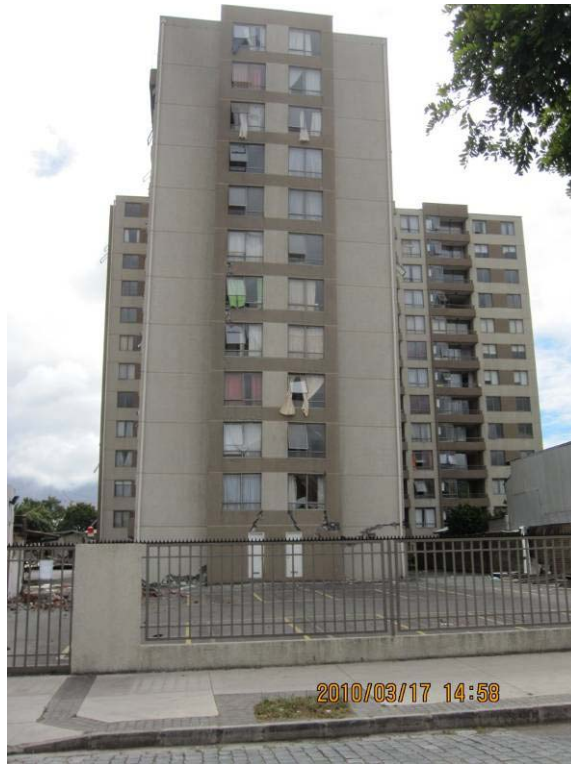
Figure 7.36. Elevation view of 1343 Salas, looking north. North wing in is the background, while the south wing is in the foreground. Note shear and horizontal cracks in the wall on first floor of south wing. (S36.8205°, W73.0619°; 1458 hrs on 03/17/10).
