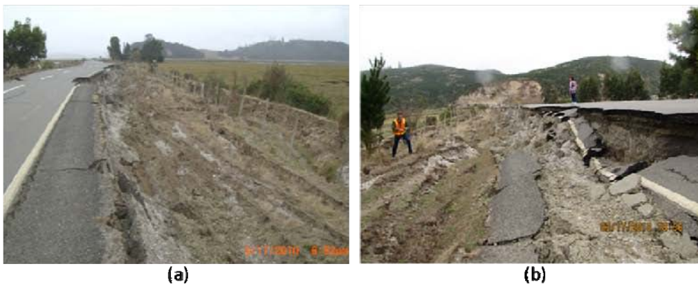
Figure 9.52. Photos showing scarps along both sides of the roadway due to bearing capacity failure in soil underlying the fill. Note lateral spreading in upper photo (S37.254161°, W73.437577° on 3/17/2010)
