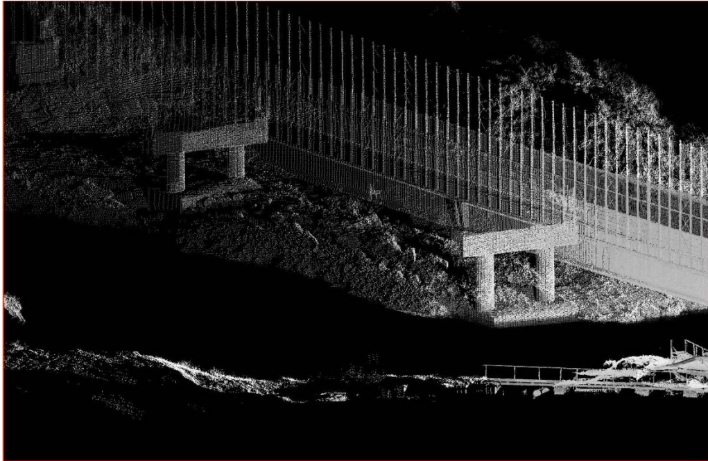
Figure 15.29. Oblique LIDAR image of Bents 2 and 3 seated in the liquefied soil mass that moved laterally to the bottom left corner.
