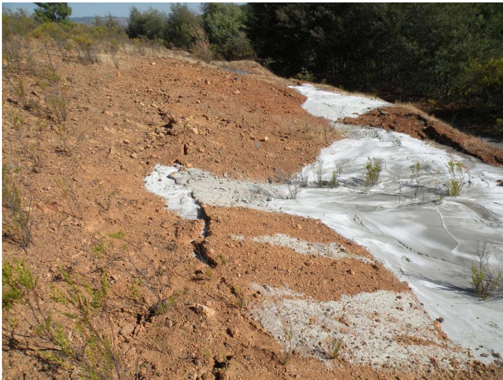
Figure 11.34. March 11, 2010. Ejecta of Tailings from Cracks Indicating Liquefaction of Tailings ( S35.183986^{\circ} , W71.761844^{\circ} )
