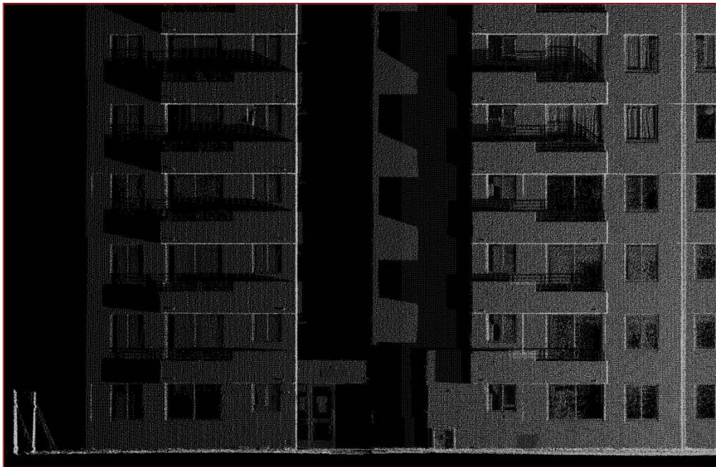
Figure 15.37. Detailed LIDAR imagery of racking of the Riesco Building (Southwest).
