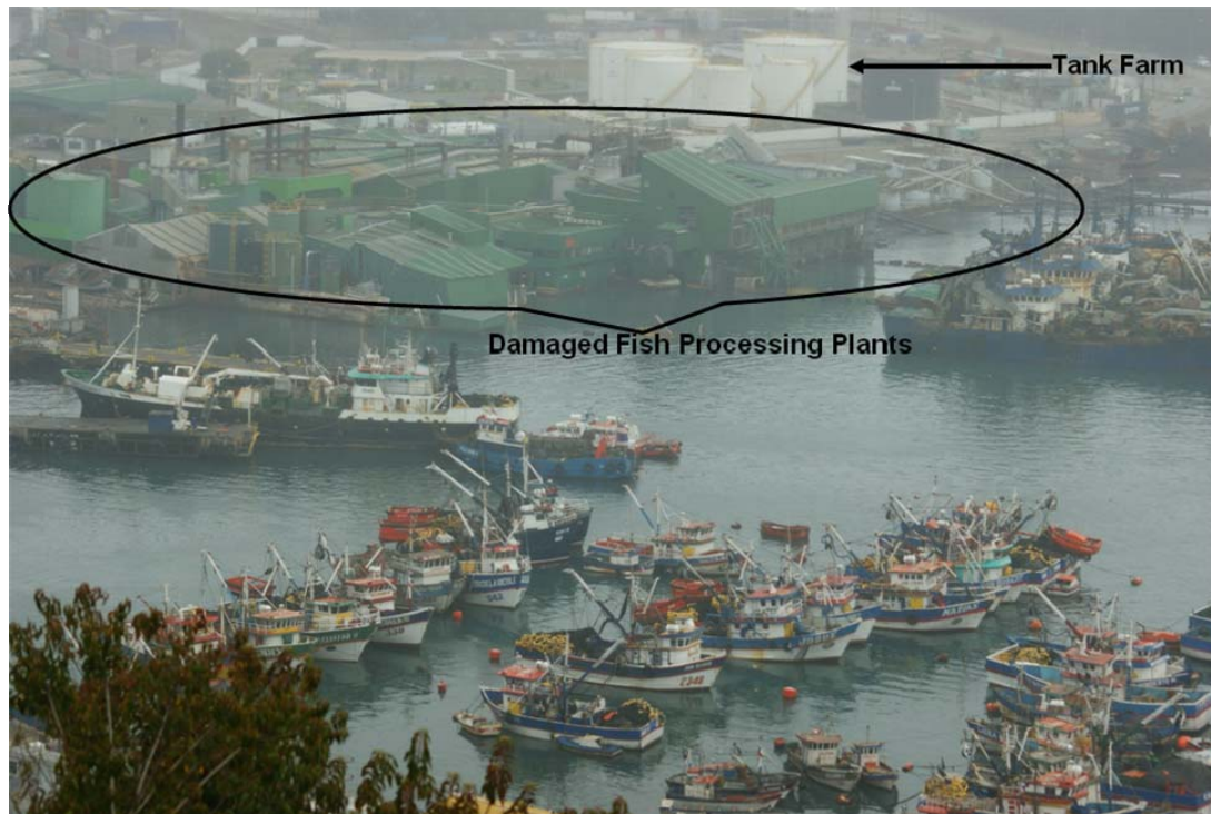
Figure 14.17. Port San Vicente, Talcahuano. View of two damaged fish processing plants and nearby tank farm. (S36.724605°, W73.136475°; 12:18 hours on 3/16/2010)
