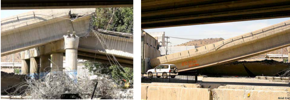
Figure 5.6. Paso Superior Lo Echevers (S33.3759° W70.7476°). Collapse of the eastbound deck of the Americo Vespucio Norte ring road (Source: http://www.flickr.com/photos/consulta_recorridos/ ).
