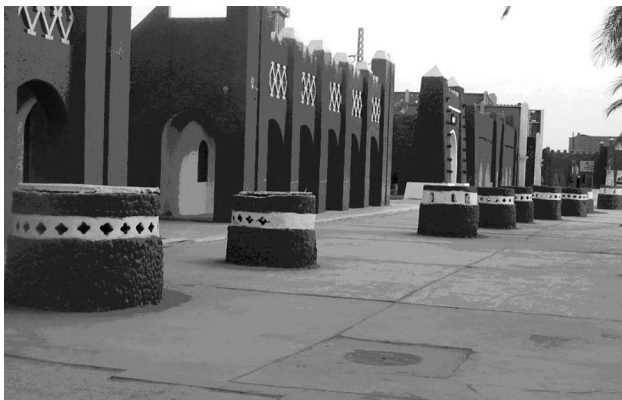
Fig. 2 Well aligned in the city center of Adrar indicator of passage of an underground gallery
