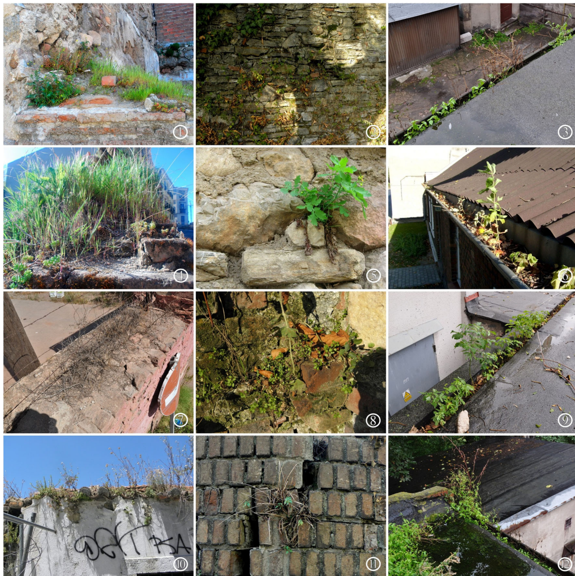
Fig. 2 Examples of Edifisols: 1 S-Av1, Avila I, Spain; 2 I-Be1, Bergamo I, Italy; 3 Pl-T4, Toruń, Poland; 4 S-Av2, Avila II, Spain; 5 R-Ri2, Rimetea, Romania; 6 Pl-T3, Toruń, Poland; 7 M-Ma1, Marrakech,
