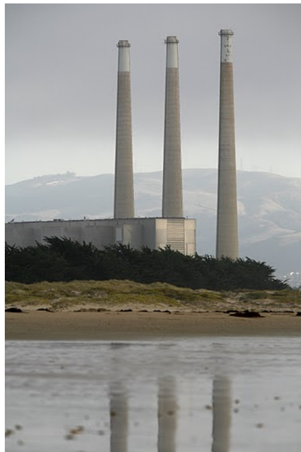
Figure 5-3 Morro Bay power plant with three 137 meter smokestacks.
