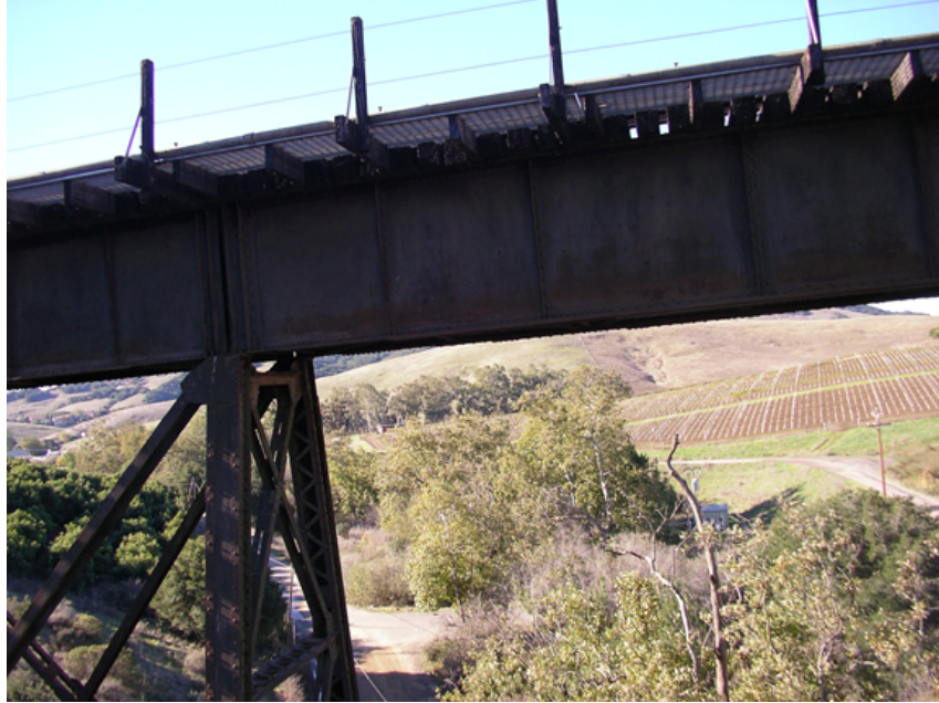
Figure 7-3 Another image with more exposed detail.
