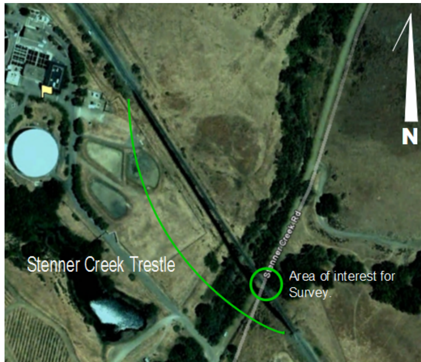
Figure 6-1 The Stenner Creek trestle with an indication of the area that was chosen for survey. Aerial picture © 2010 Google Earth.
