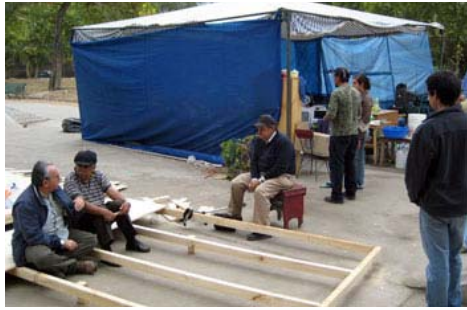
Cal Poly professor William Siembieda (far left) speaks with Chilean residents who were forced from their homes by earthquake damage and set up temporary residences nearby.
