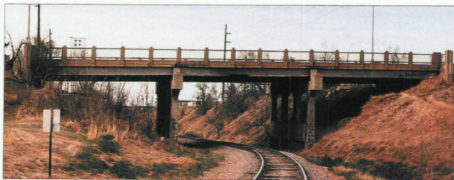
Fig. 1: Colorado State Highway Bridge E-17-AH
