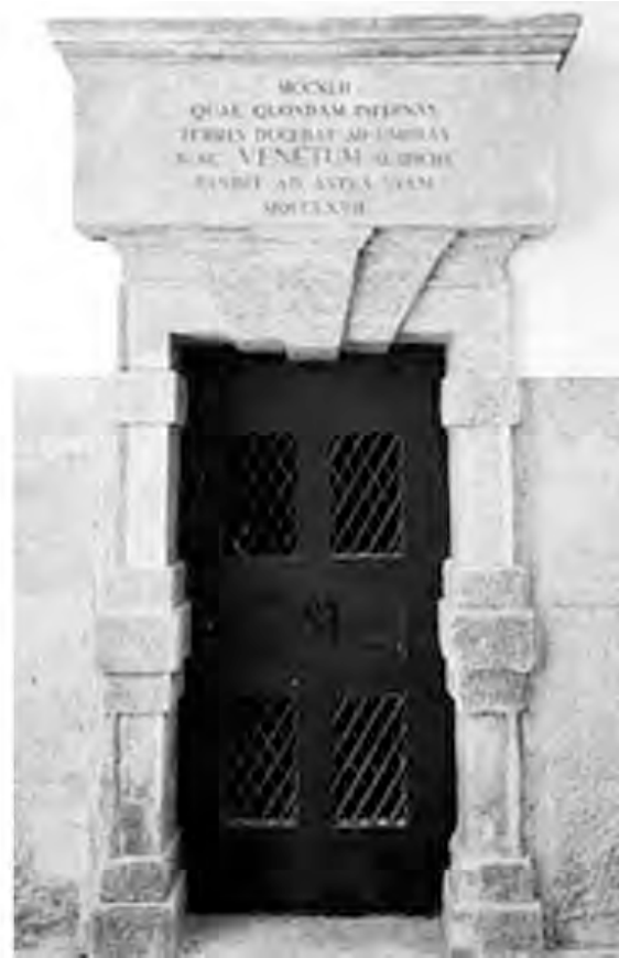
figure 18 Door frame at La specola, Cerato
