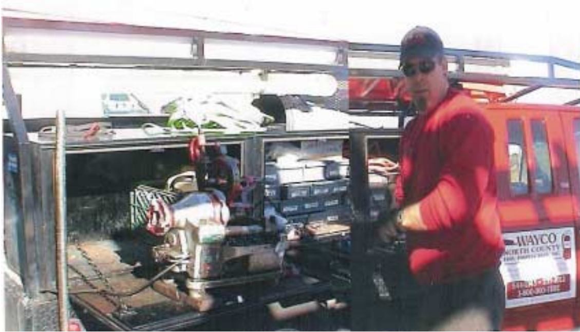
Figure 13 Threading Steel Pipe
