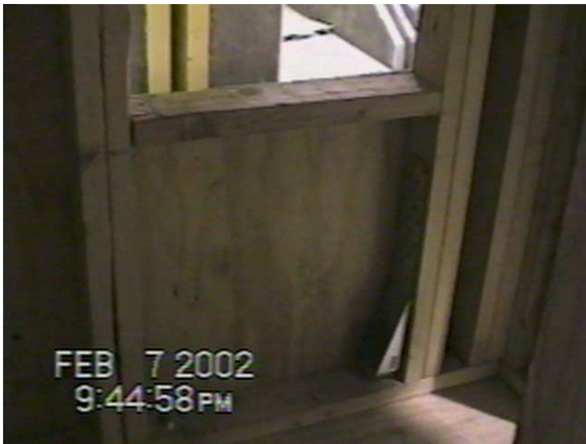
Figure 8 View of a hold-down from inside.
