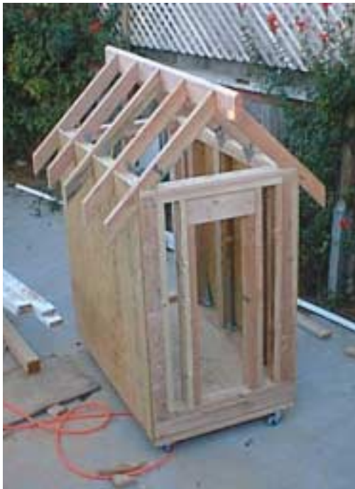
Figure 5 Picture of Partially Completed Model
