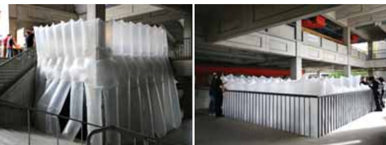
Figure 10: Final installation in the architecture building's stair court, views from the first and second levels.
