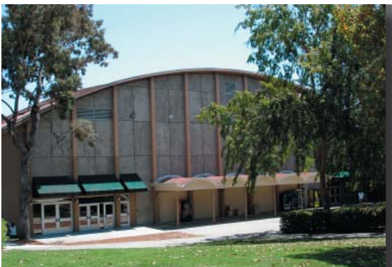
Mott Gym HID saves over 200,000 kWh per year.
