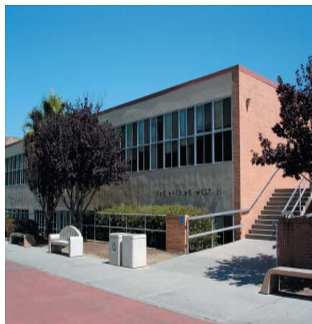
One of only three CSU campuses to take advantage of a systemwide program, Cal Poly installed photovoltaic panels on Engineering West in 2006.
