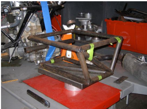
Figure 5.6: Rear box aligned with the existing frame and engine
