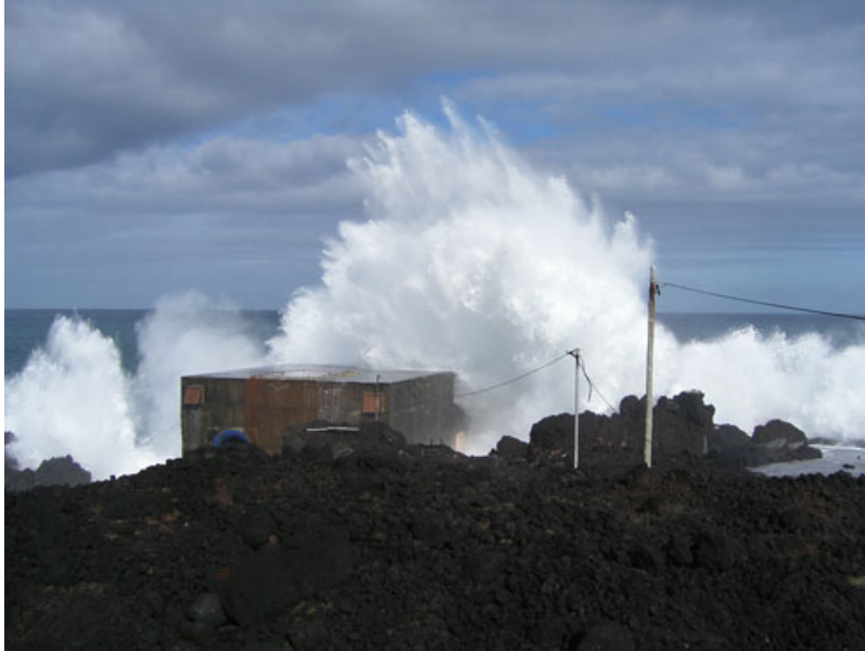
Figure 8. Oscillating water column wave energy converter at the European Wave Energy Center, on the island of Pico, Portugal.
