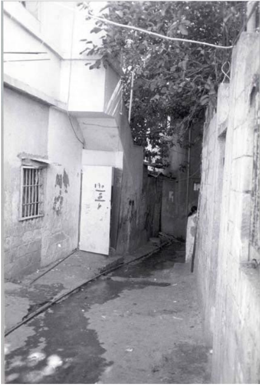
Figure 3.1: Water pipes in the right of way in Mar Elias.
