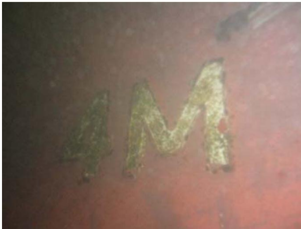
The starboard vertical side at 4 m bow mark.
