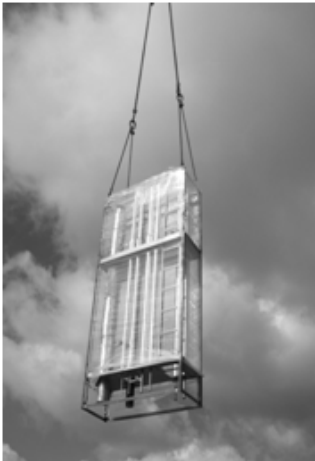
Figure 1 The prefabricated shaft
