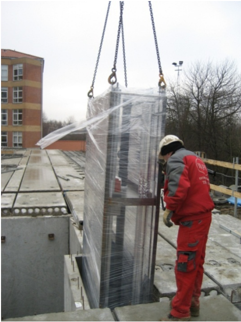
Figure 4: Installation of the NCC Shaft
