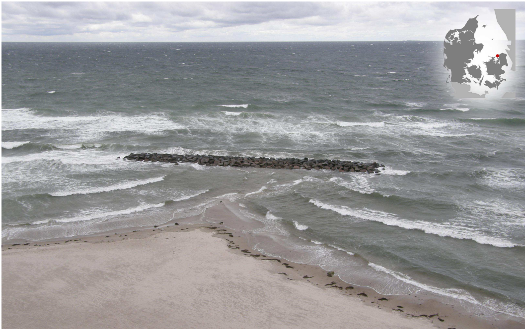
Figure 1.3: Salient in the lee of a shore parallel detached breakwater at the North coast of Sealand, Denmark. Photo by Jens Kirkegaard, August 2011.
