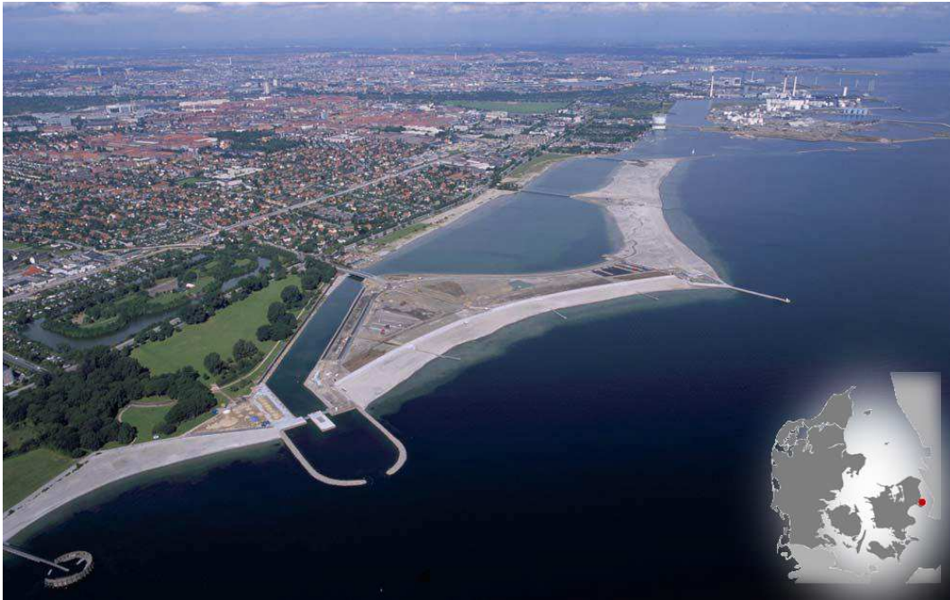
Figure 1.4: Aerial photo of Amager Beach Park, Denmark. Single long groynes may be used to divide a beach into smaller sections. The photo from Mangor et al. (2008).
