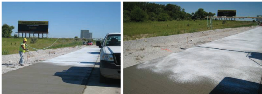
Figure 4.18 Concrete surface after spraying with the concrete curing compound.
