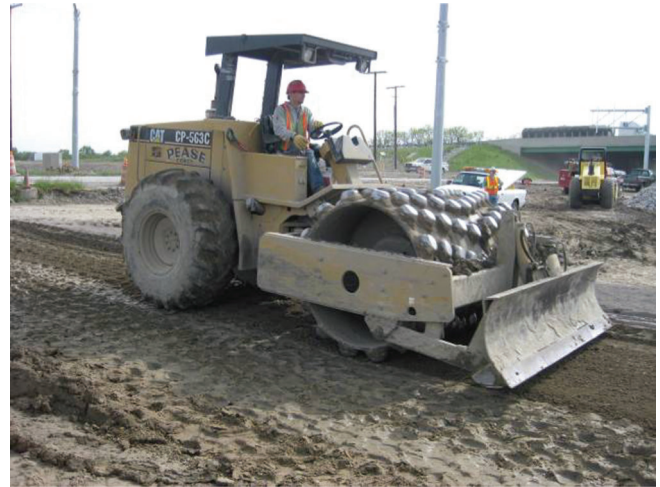
Figure 4.7 Compaction of the subgrade with sheepfoot roller.
