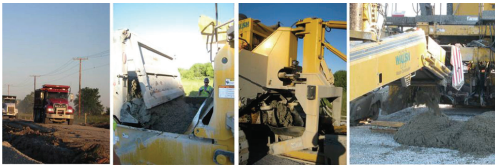
Figure 4.14 Preparation and pouring of concrete pavement.
