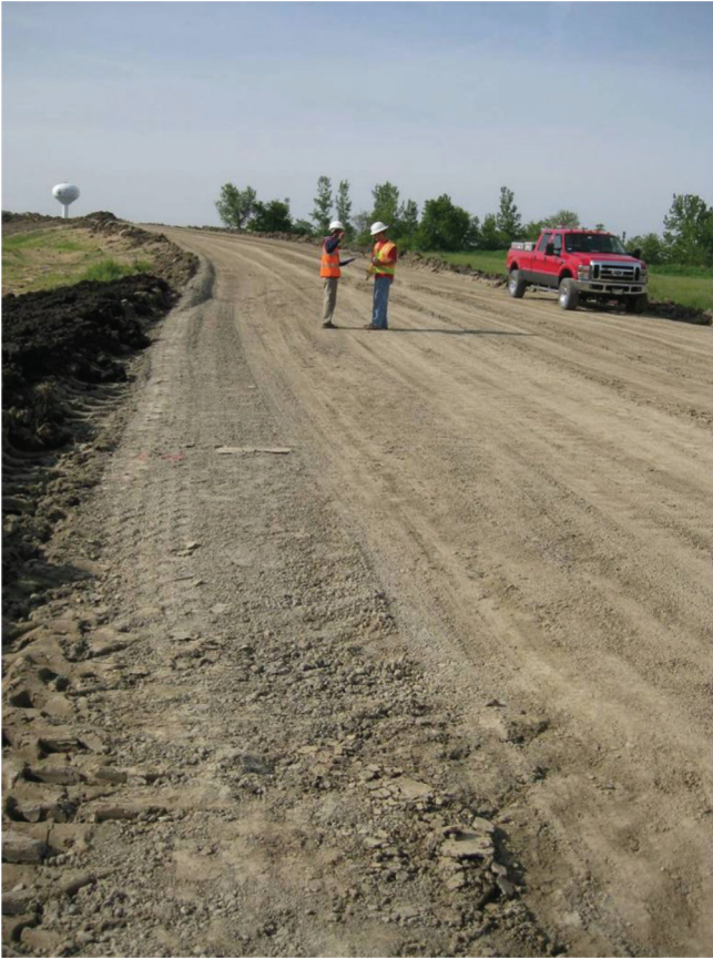
Figure 4.1 In situ subgrade soil of the SW ramp before soil stabilization.
