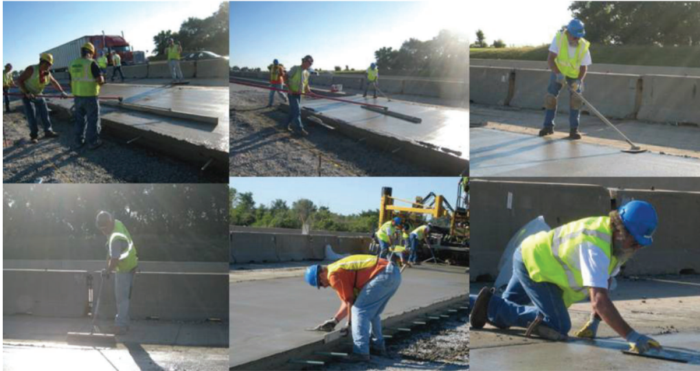
Figure 4.16 Final leveling of the concrete surface.
