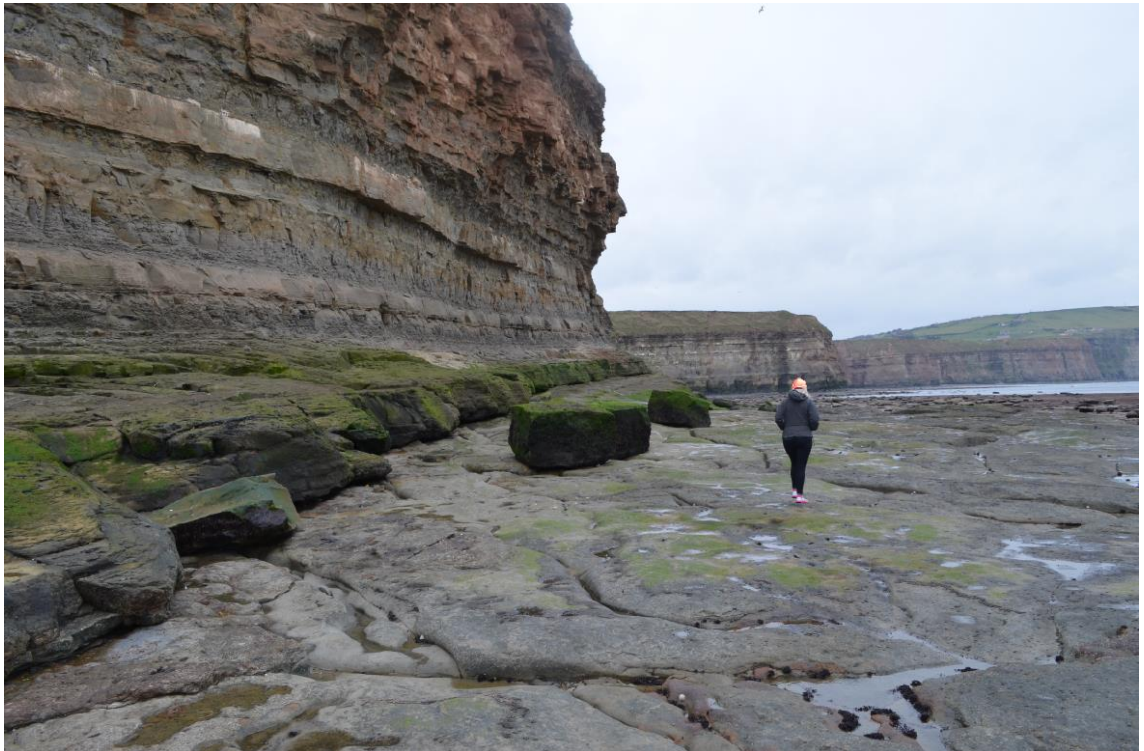
Figure 3.7: Cliff toe and face at Site 2 with fieldworker for scale. Note the cliff toe shelf extending approximately 12 m seawards from the vertical cliff face. Image was taken prior to scanning commencement and large boulders in foreground were not present during the study period.
