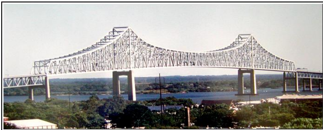
Figure 1-2 Commodore Barry Bridge
