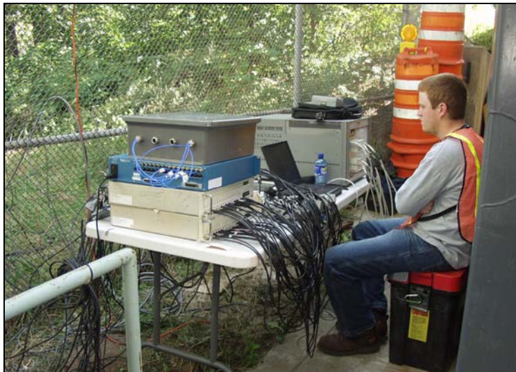
Figure 5-13 Data acquisition system at the Henry Hudson Bridge
