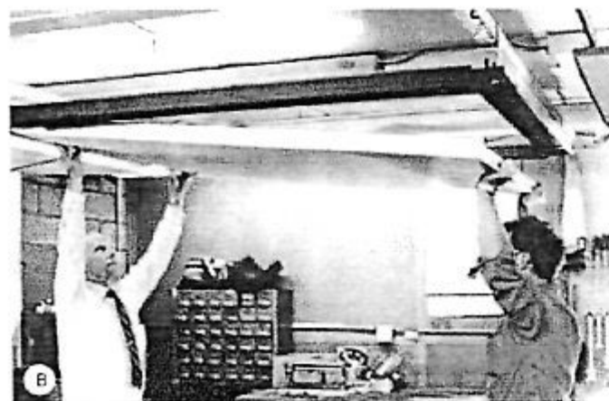
A. Mockup to demonstrate integration of services and accessibility for IAC Mark I Noise-Lock® Ceiling for Philip Morris. B. Mockup depicting downward accessibility of 60 in. x 66 in. (1524 mm x 1676 mm) ceiling modules weighing 70 lb (32 kg) for AT&T. C. Mockup of interspatial load bearing IAC Mark IV Noise-Lock Ceiling module, 48 in. x 60 in. (1219 mm x 1524 mm)
