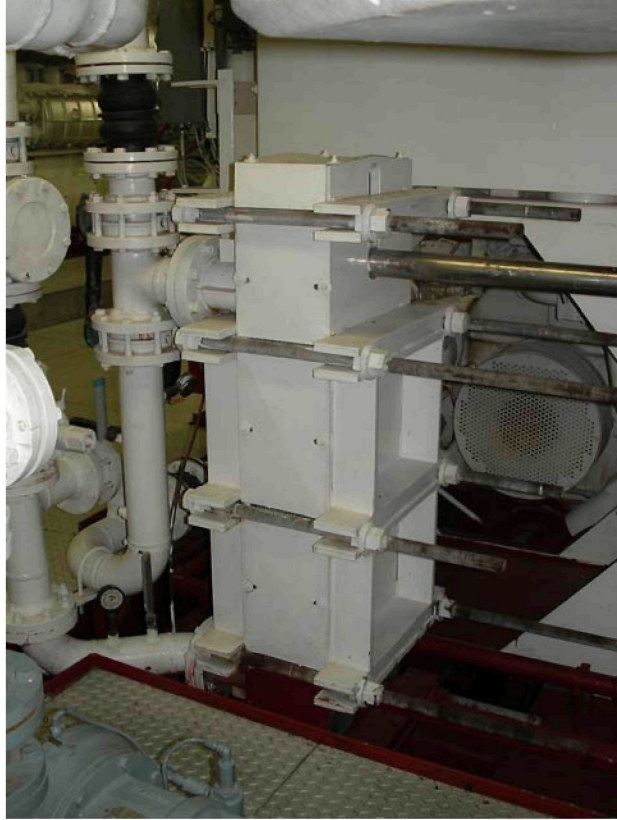
Figure 1. Typical Main Engine Plate Heat Exchanger
