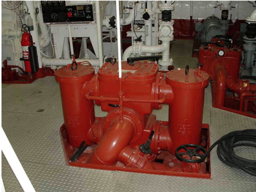
Figure 2a. Typical Duplex Strainer (Side View).
