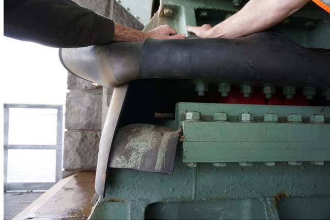
Figure 7. Bridge bearing protection
