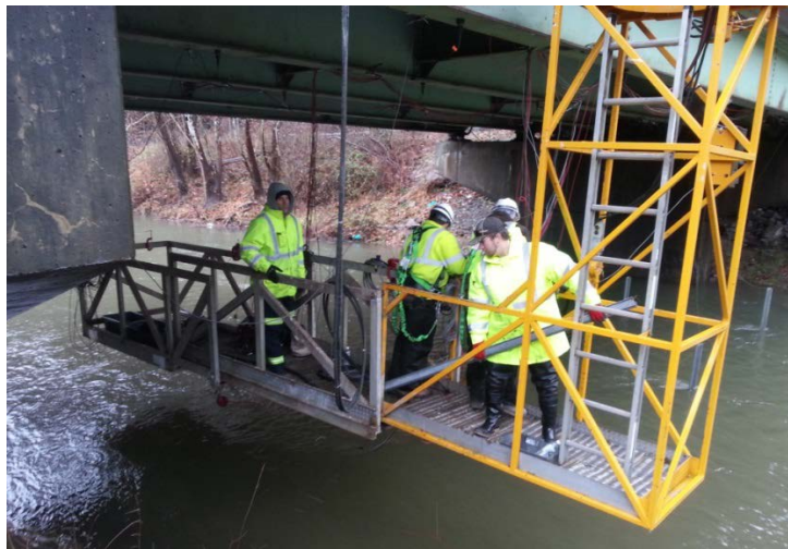
Figure 7-60: Underside Installation with Hydra Platform
