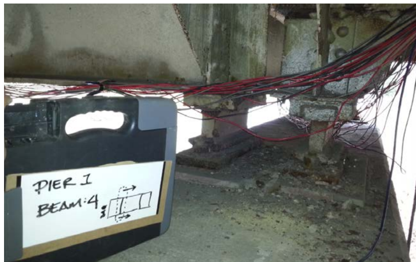
Figure 6-7: Expansion Bearing at Interior Girder – Pier 1
