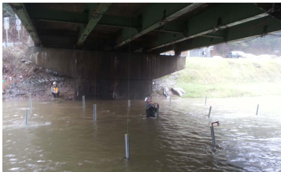
Figure 7-50: Installation of String Pot Displacement Sensors
