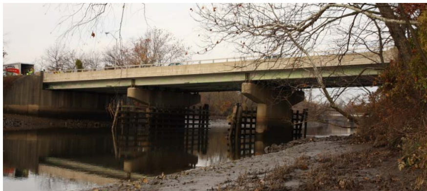
Figure 5-5: Pennsauken Creek Bridge in Palmyra, New Jersey – Elevation View
