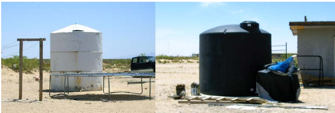
Figure 2: Metallic and HDPE water storage tanks used by residents of Las Colonias
