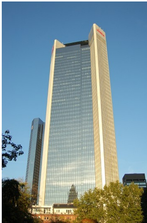
Figure 2.1. The Trianon in Frankfurt constructed 1990-1993 was the first high-rise building incorporating HSC in Germany (structurae, 2019a).
