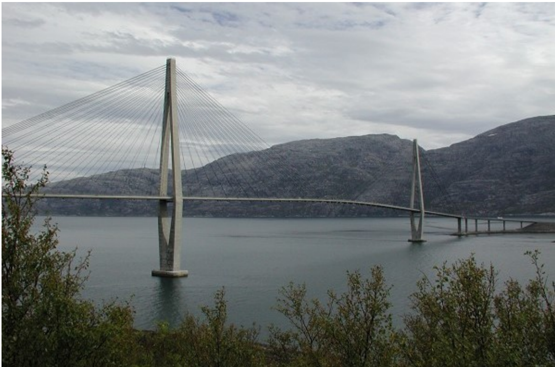
Figure 2.2. The cable stayed Helgeland Bridge in Norway (structurae, 2019b).
