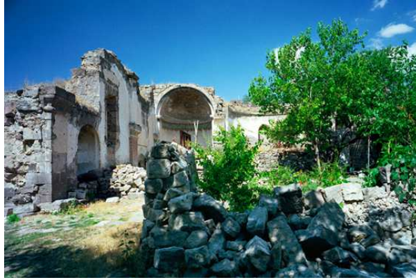
Fig.13 Germir Surp Toros Church current condition 225
