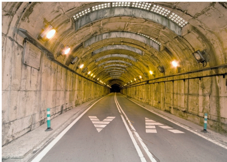
Figure 1. Upper windows to use natural light in an almost closed tunnel in Bielsa (Spain) (Image bought in www.istockphoto.com ).
