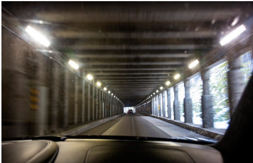
Figure 2. Lateral columns to use natural light in an almost open tunnel (Spain) (Image bought in www.istockphoto.com ).
