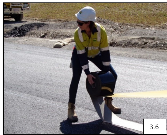
Figures 3.3 – 3.8: Manual roll-out of Bitac®, Manual wind-up of tape backing, Unpacking tape, A group participatory ergonomics workshop on-site, and Investigator task trial
