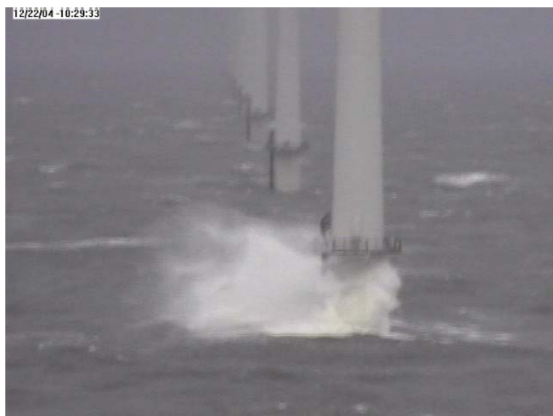
Figure 1.7: Severe impact of the roller on an offshore wind turbine. From Nielsen et al. (2008).
