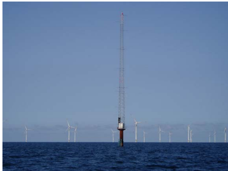
Figure 2-3. Photograph of the 62 m tall meteorological mast M2 at Horns Rev, erected in 1999. The mast position 2 km to the north of the wind farm is indicated in Figure 2-2. Photo courtesy Paul B. Sørensen, Elsam Engineering A/S.
