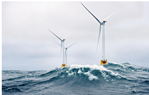
Figure 1.2: Example of an offshore wind farm, Block Island, USA [5]
