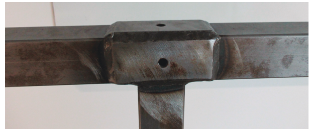
FIGURE 12: Close-up of the center of the T structure from Figure 10.
