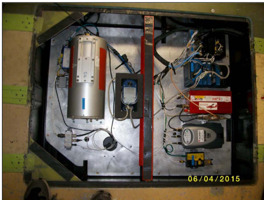
Figure 3: Instrument installation in the camera bay below the floor in the Twin Otter cabin; ALS (left), OxTS INS (middle right) and Trimble GPS receiver (lower right). Note ALS and OxTS INS axis are mounted along aircraft centre line.
