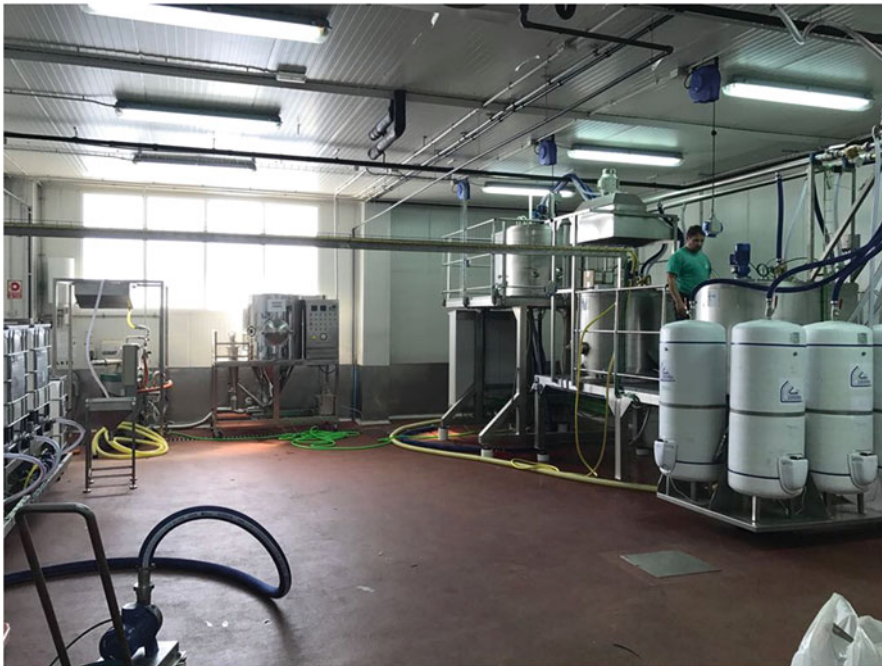
Fig. 17.5 iDVP3 located in the Port of Marín (Spain)
