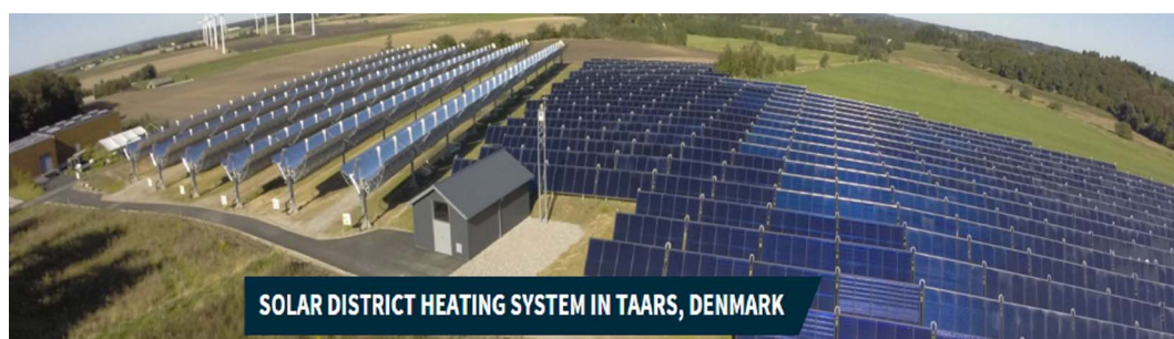
Fig. 2. Picture of the Taars solar heating plant.
