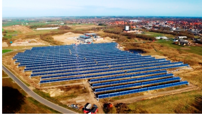
Fig. 9 The parabolic trough collector array in Brønderslev, Denmark (Source: Aalborg CSP A/S).
