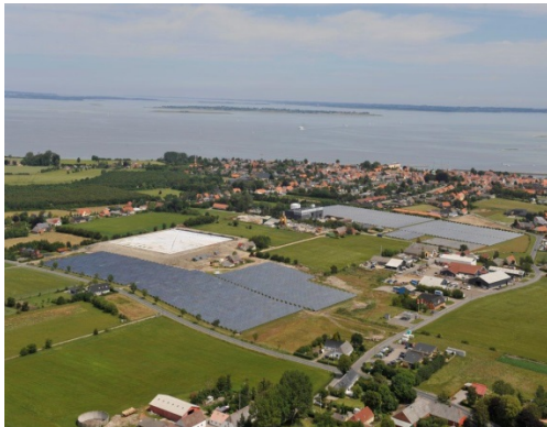
Fig. 2a Marstal plant (33300 m 2 )
