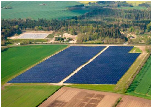
Fig. 2b Dronninglund plant (37573 m 2 )
