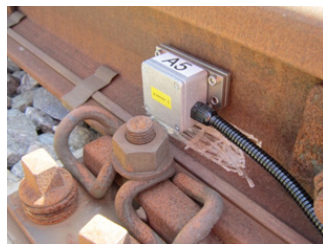
(b) Accelerometer A5 magnetically connected to the rail web
