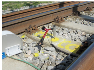
(c) Displacement sensor resting on the sleeper
