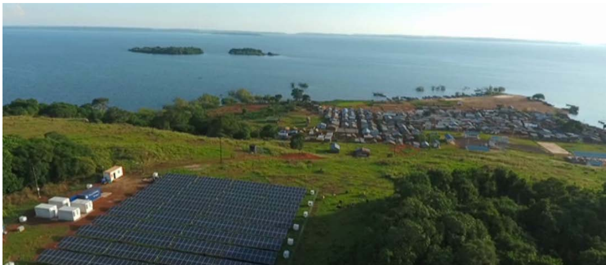
Figure 3. The 228 kWp installed solar mini-grid project on Kitobo Island, Lake Victoria, providing electricity to 520 domestic and business users.
