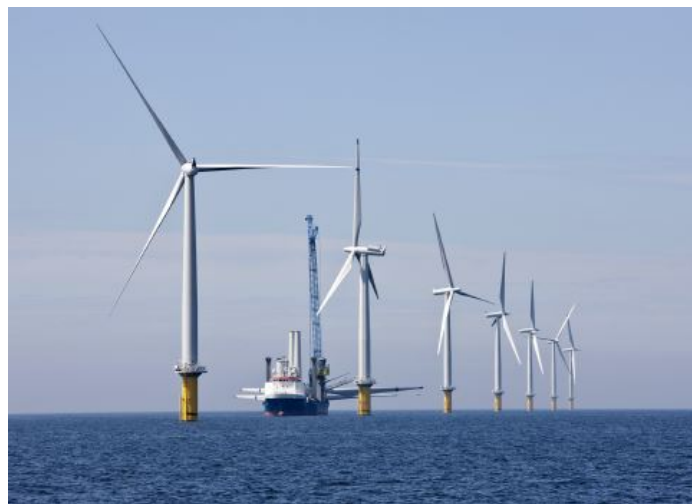
Figure 1.1: Offshore wind turbine park, under construction (Energy efficiency and renewable energy).
