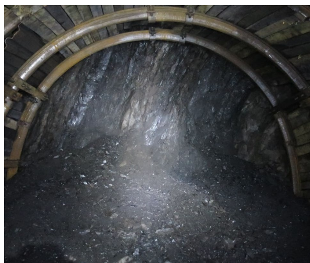
Fig. 3 Sublevel development heading in Seam #8 illustrating the friable nature of the coal seam
