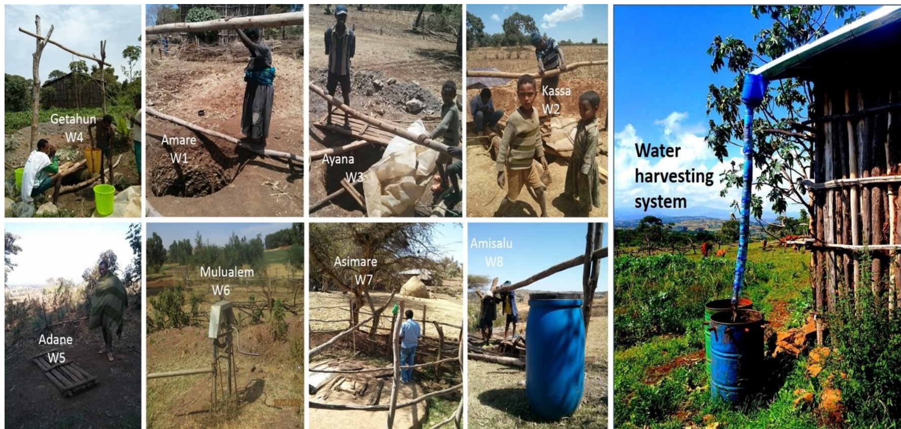
Figure 5.2: Photos of the 8 water table height monitoring wells (W1–W8), and water harvesting system installed for experiment. Photo of W6 was taken in 2015 before it was opened (during data collection, it was opened while its depth reduced from 11 m to 2.3 m due to the sliding down of the soil).
