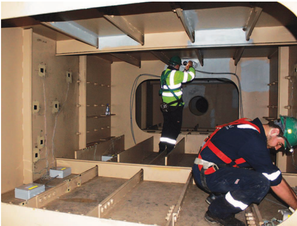
(c) Steel box girders of A380 Thame Valley Viaduct (MISTRAS group, 2017).
