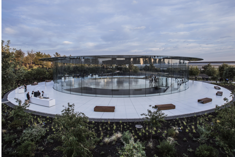
Figure 1.1: The Steve Jobs Theater in the Apple Campus in California, United States with the world's largest carbon fiber roof (Martin, 2017).
