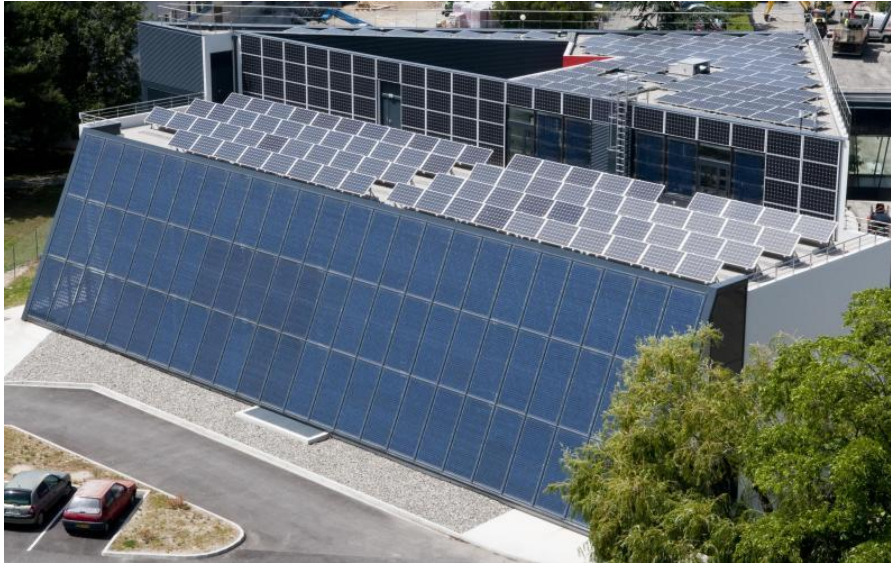
Figure 2.25 ADREAM building of the LAAS-CNRS
