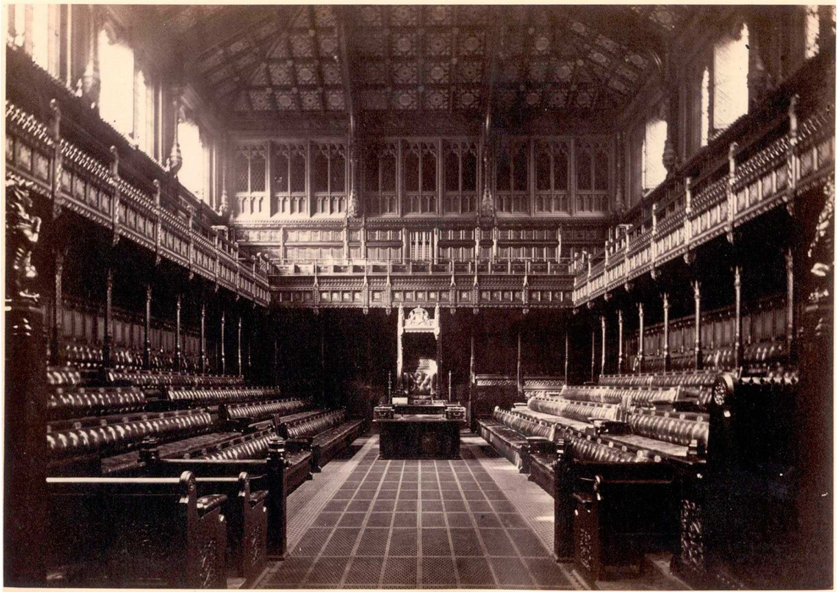
Figure 7. House of Commons debating chamber, 1868, showing the windows opened to ‘flush’ the chamber with fresh air. Source: Harrington (1869, plate IX).
