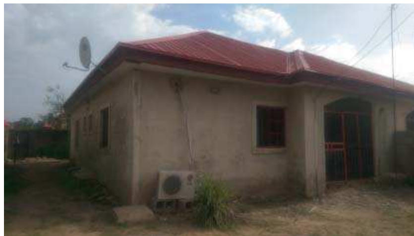
Figure 4.17: LGH2AC in Lugbe, Abuja, showing the main building.
