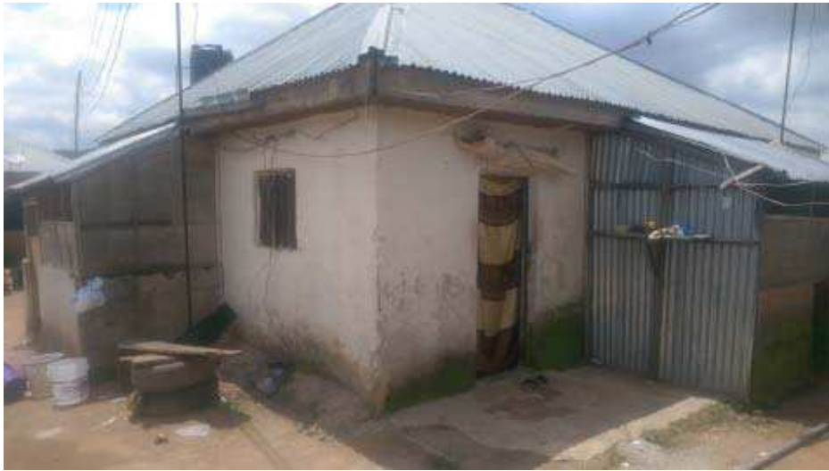
Figure 4.24: MPH2NV at Mpape, Abuja, showing the main building.
