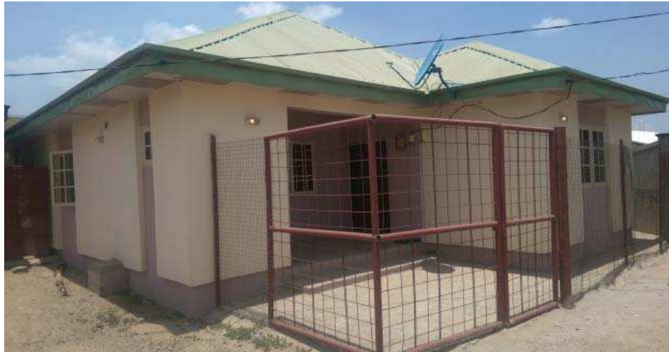
Figure 4.42: BWH2AC at Bwari, Abuja, showing the main building. Source: researcher's survey, 2015
