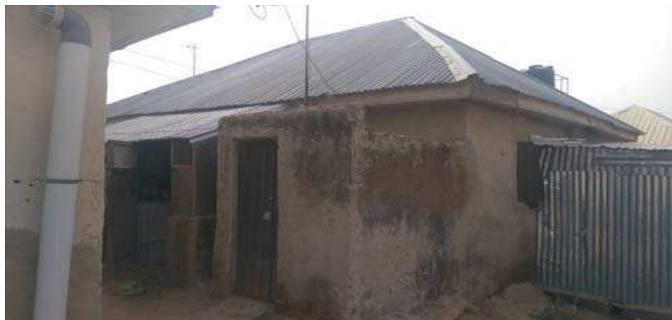
Figure 4.21: MPH1NV at Mpape, Abuja, showing the main building.
