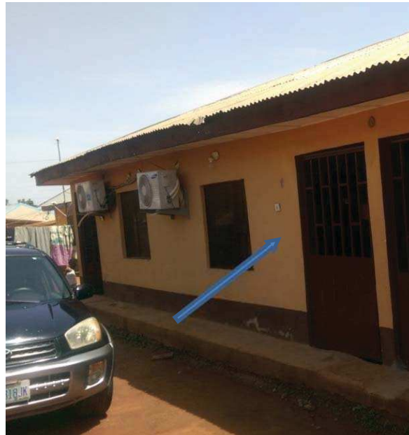
Figure 4.30: DAH2 at Dutse Alhaji, Abuja, showing the main building.
