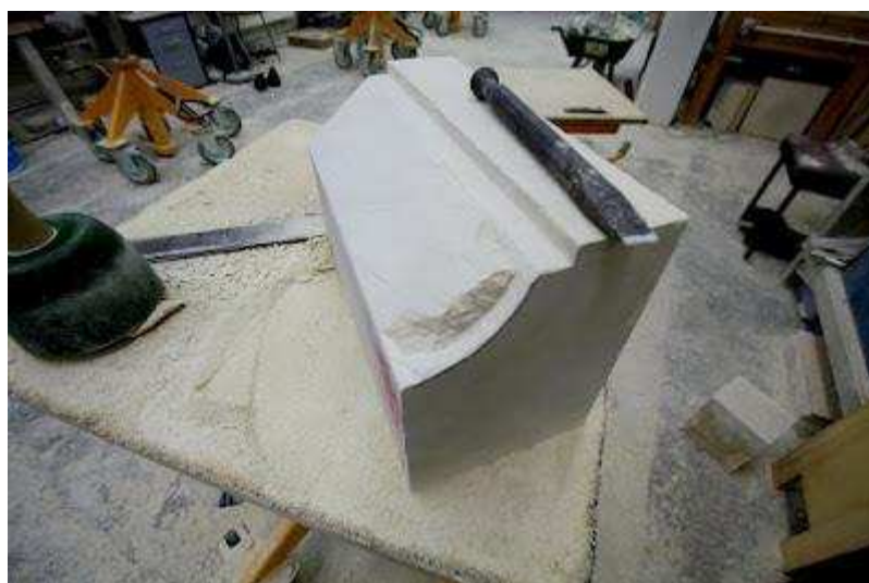
[Figure 4-16 The drafting chisel was used to cut along the curved moulding profile. Photo by the author.]
