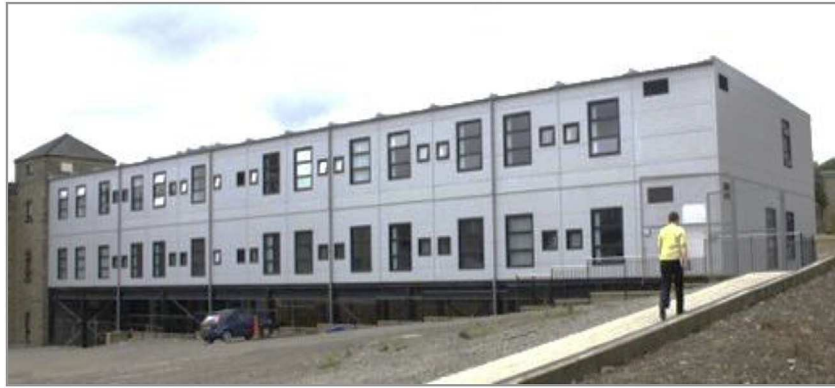
Fig. 2. The East facing façade of the 2008 modular building at Bradford Royal Infirmary.
