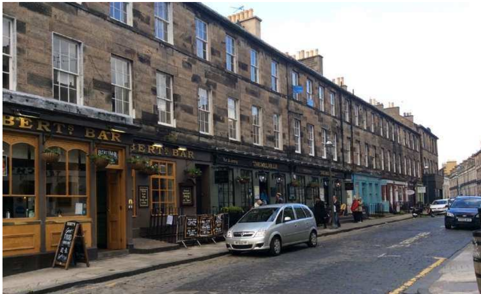
Figure 38: Example of ashlar-faced architecture in the New Town of Edinburgh. © Francesca Giliberto
