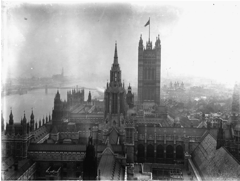
Fig 11. Aerial view of the Houses of Parliament (looking eastwards) showing the position of local ventilation shafts introduced by Reid and Barry after abandoning the central up-cast shaft in 1846, c 1900, PED: Farmer 743. Photograph: © Parliamentary Estates Directorate.
