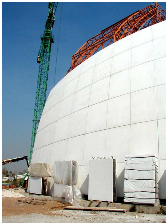
Fig. 4 The smaller shell after its completion. At its bottom some ashlar ready to be assembled for the medium-size shell. (Picture by the author, taken 04/04/2001).
