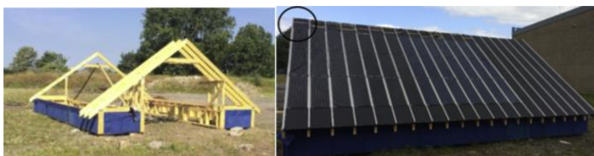
Figure 20. The heat mats' based solar roof installation [42].
